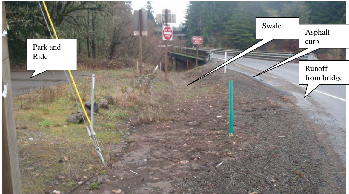
Photo 1: Biofiltration swale. Willamina – Salem Highway is to the right
