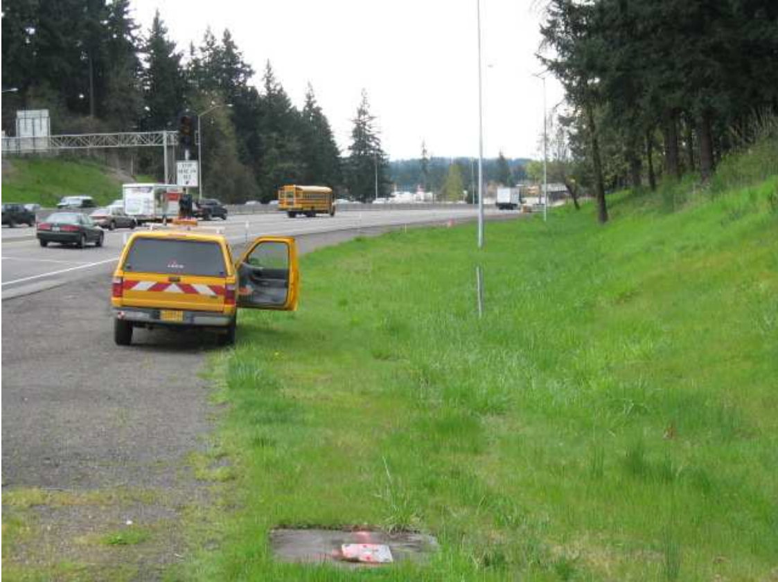
Photograph 1 Existing swale looking south. The proposed swale will shift to the east with the reconstructed onramp.
