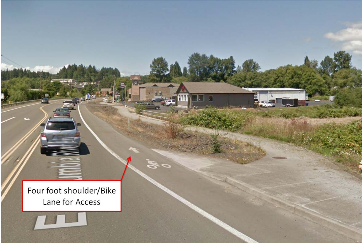
Figure 4: Four foot shoulder/bike lane, facing west from US30
