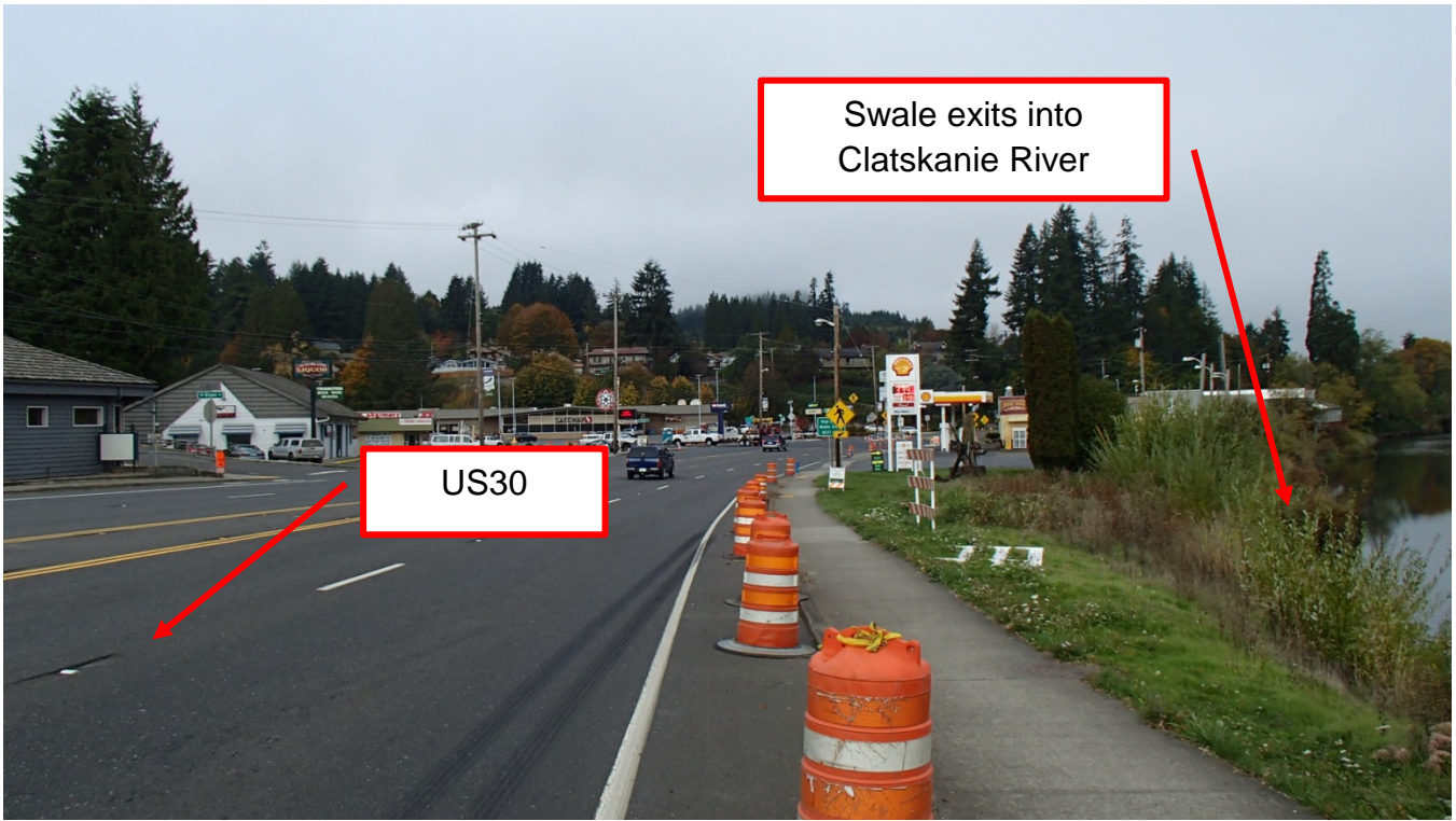
Photo 1: A view of swale and outlet into Clatskanie River, looking northwest along US30
