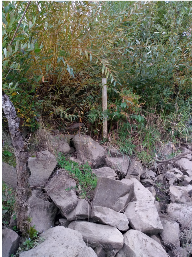
Photo 2: Swale outlet into Clatskanie River, looking west
