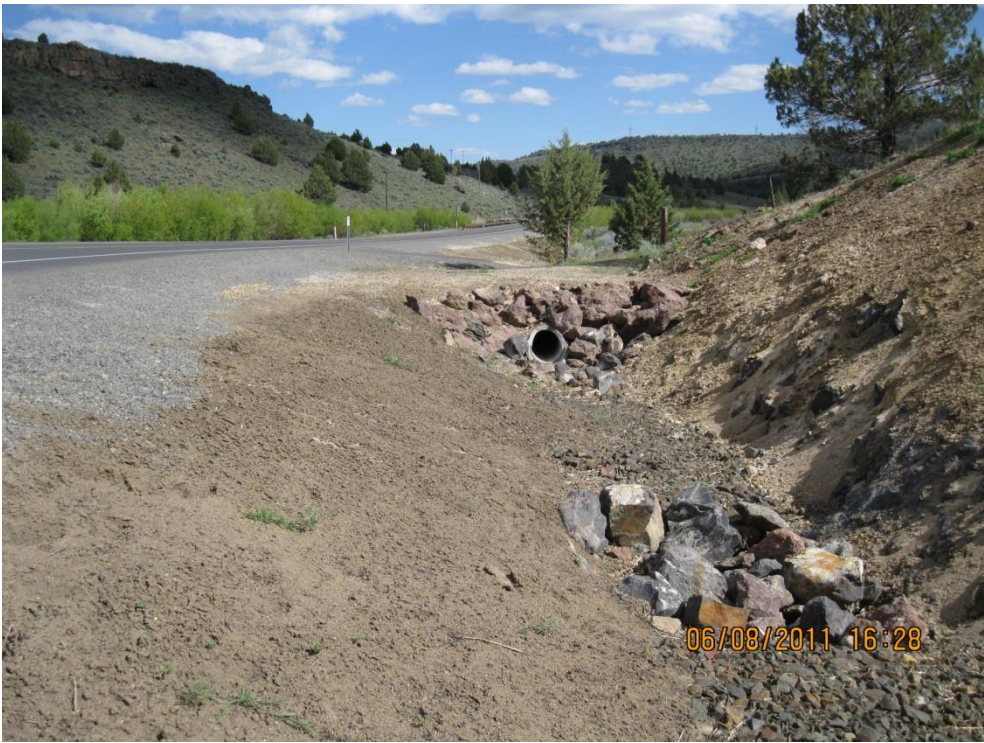
Figure 1: DFI No. D00522, looking southeast
