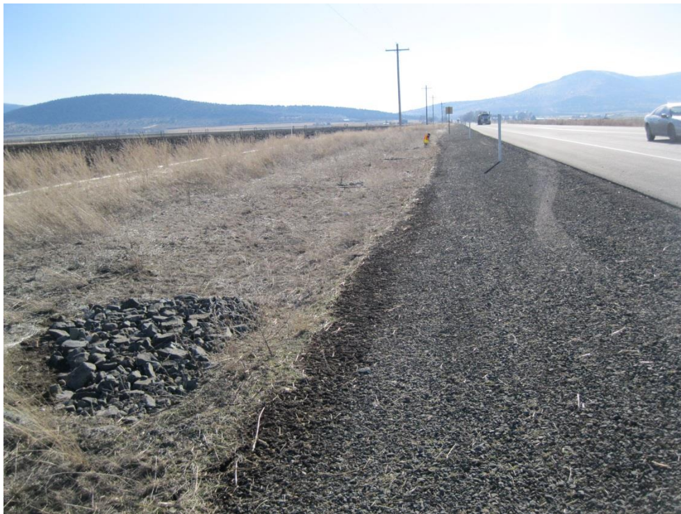
Figure 1: DFI No. D00485, looking south
