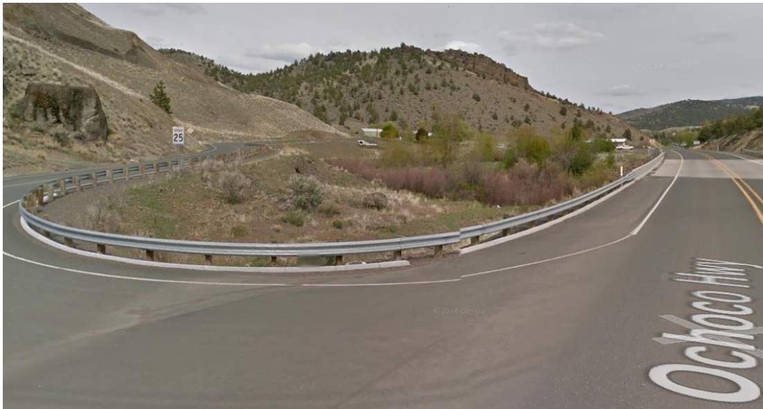
Figure 3: Surrounding guardrail limits maintenance access to the facility location.
