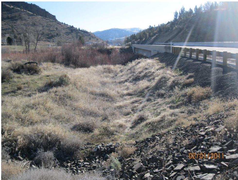
Figure 1: DFI No. D00473, looking southeast
