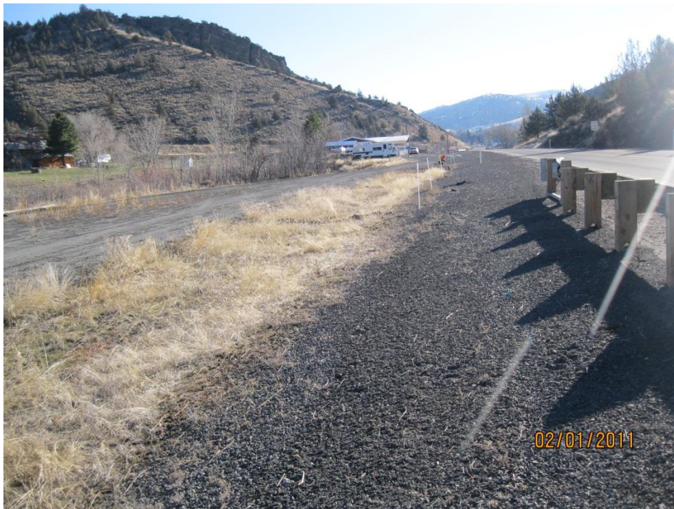
Figure 1: DFI No. D00472, looking east
