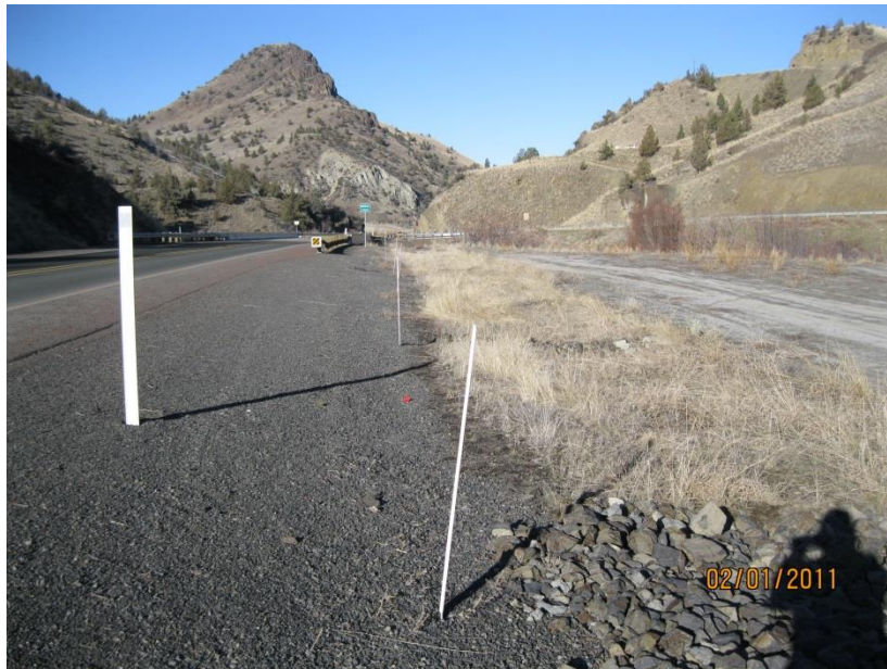
Figure 3: Roadside shoulder on Ochoco Hwy looking west
