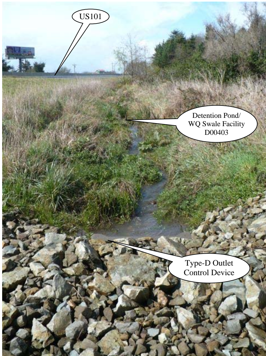
Photo 2: Looking north, stormwater is flowing from the top of the picture towards into the outlet control device, shown. During High flow events stormwater will be detained in the pond and released at a controlled rate through a 6-inch pipe located in the Type-D inlet.
