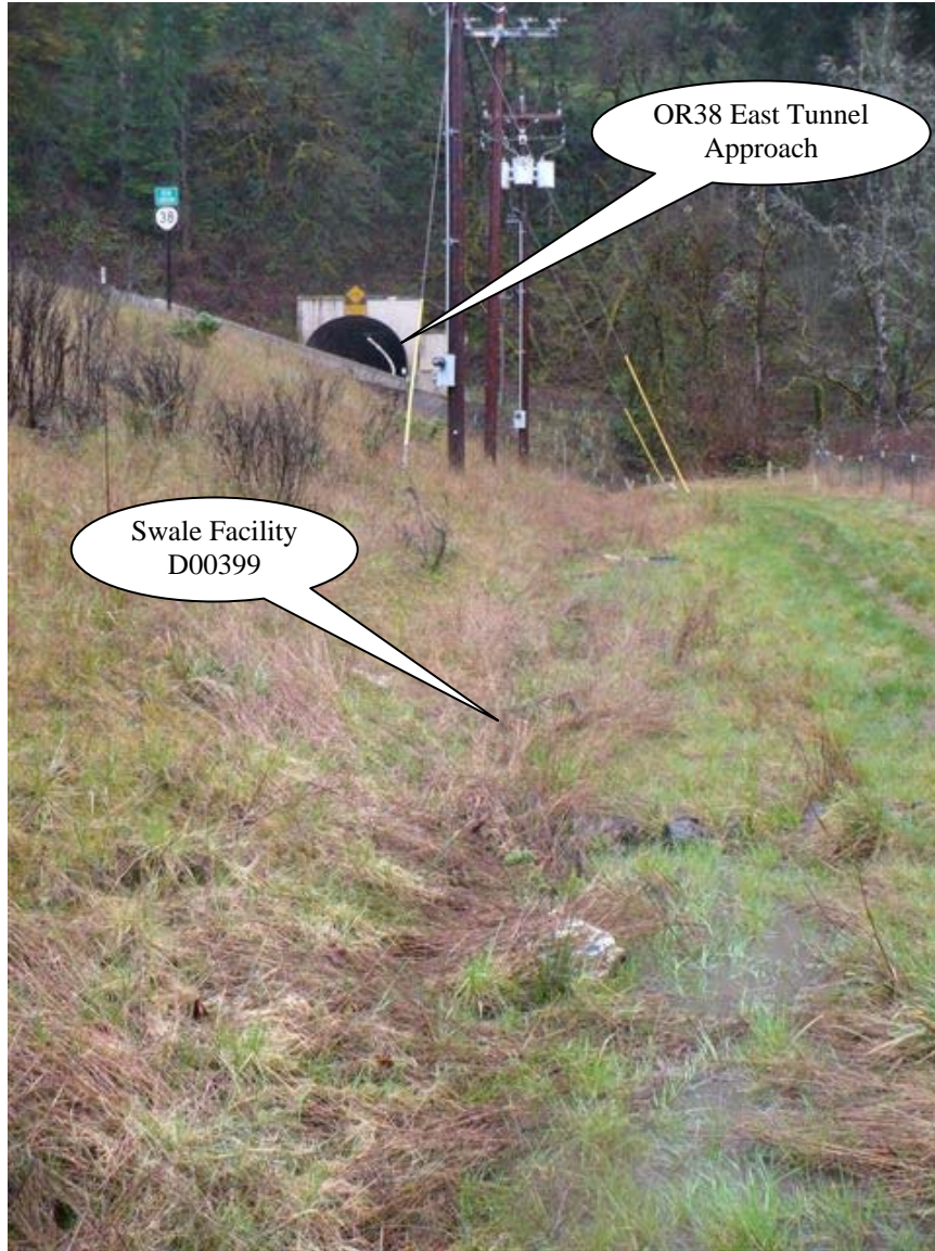
Photo 1: Looking west, storm flow generated from OR38 on the left side of the picture contributes stormwater into the swale. Stormwater is flowing from the bottom of the picture towards top of the picture.
