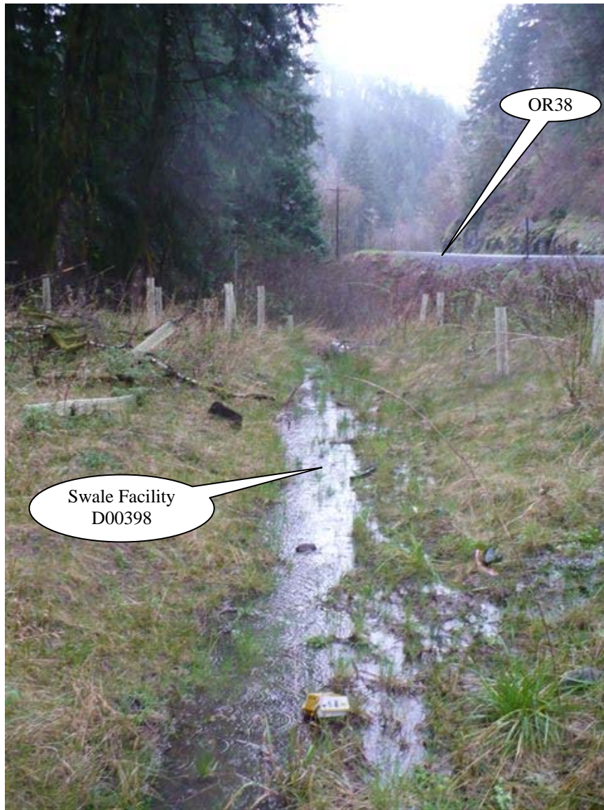
Photo 1: Looking west, storm flow generated from OR38 on the right side of the picture contributes stormwater into the swale. Stormwater is flowing from the bottom of the picture towards top of the picture.
