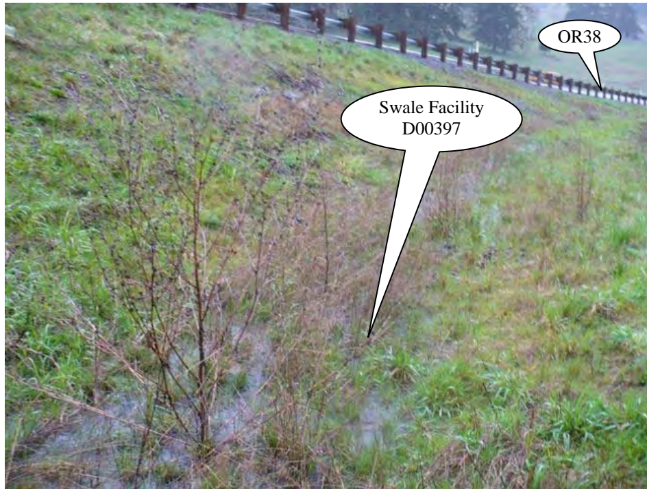
Photo 3: Looking east, storm flow generated from OR38 on the left side of the picture contributes stormwater into the swale. Stormwater is flowing from the top of the picture towards the bottom of the picture.
