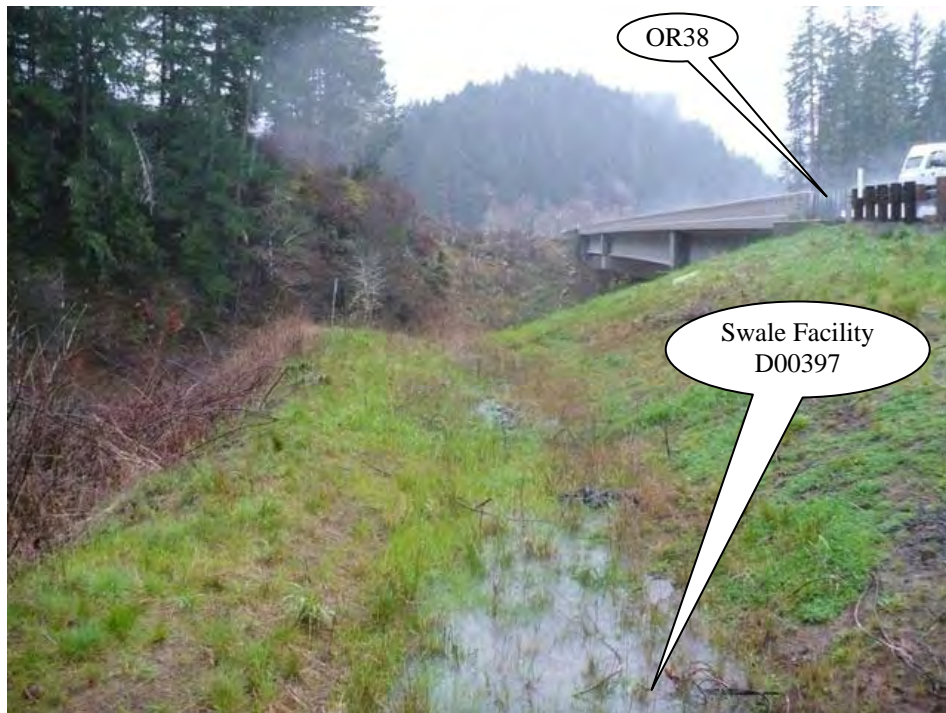
Photo 2: Looking west, storm flow generated from OR38 on the right side of the picture contributes stormwater into the swale. Stormwater is flowing from the bottom of the picture towards Elk Creek at the top of the picture.
