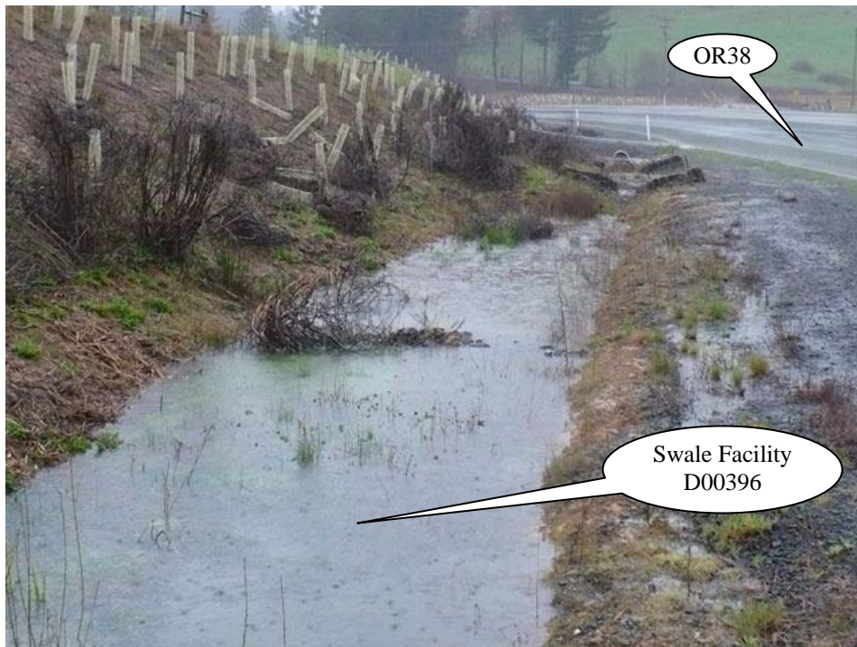
Photo 2: Looking east, storm flow generated from OR38 on the right side of the picture contributes stormwater into the swale. Stormwater is flowing from the bottom of the picture towards the top of the picture.
