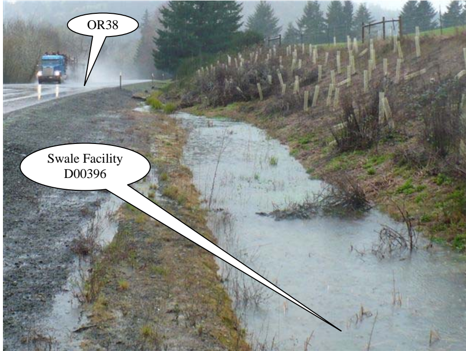
Photo 1: Looking west, storm flow generated from OR38 on the left side of the picture contributes stormwater into the swale. Stormwater is flowing from the top of the picture towards Elk Creek at the bottom of the picture.
