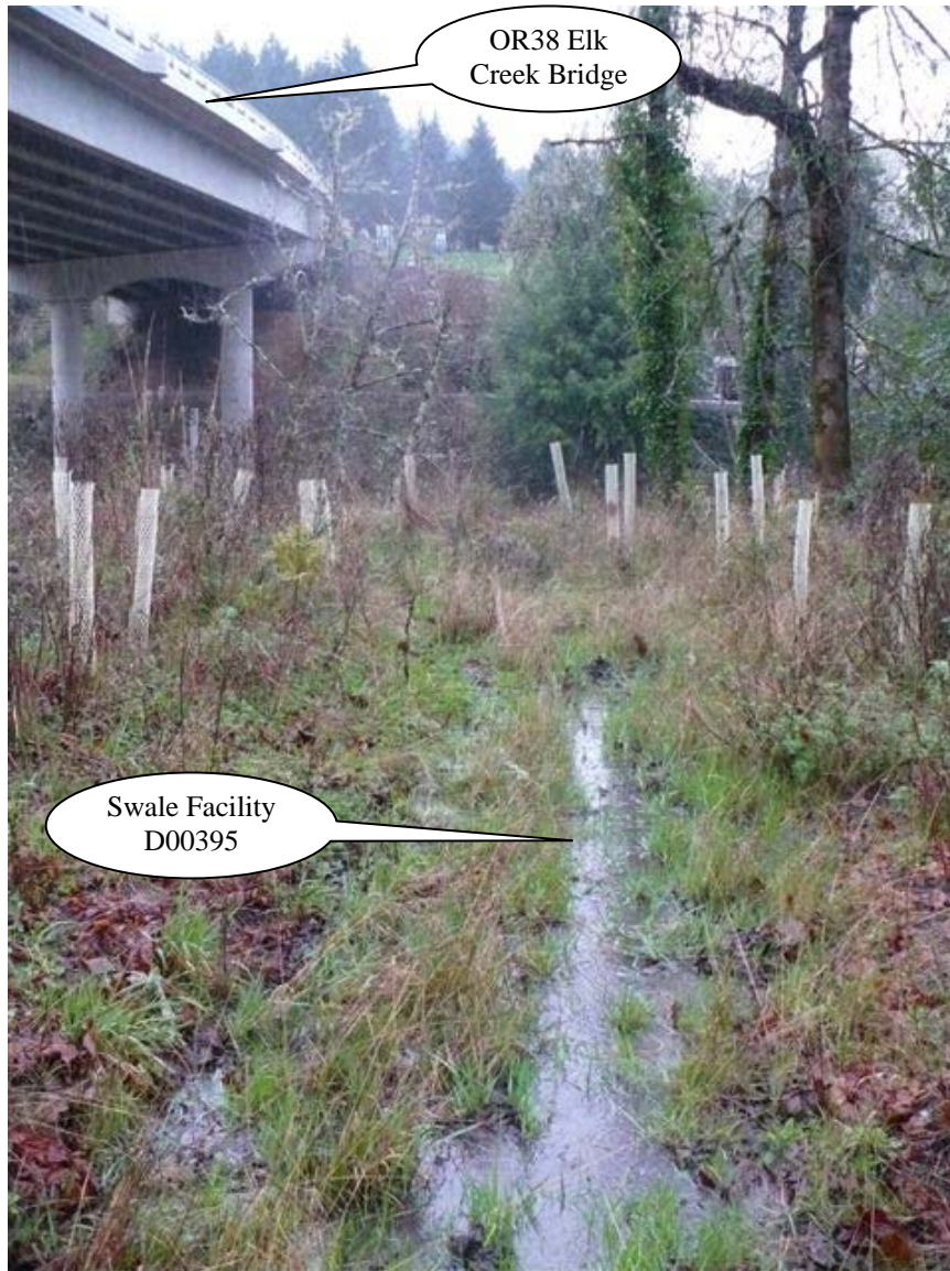
Photo 1: Looking east, storm flow generated from the Elk Creek Bridge on the left side of the picture contributes stormwater into the swale. Stormwater is flowing from the bottom of the picture towards Elk Creek at the top of the picture.
