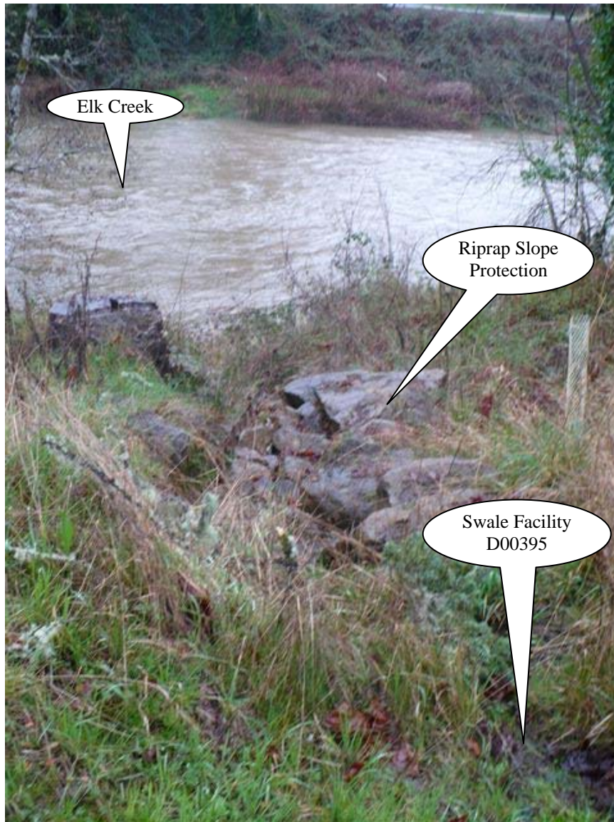
Photo 2: Looking east, stormwater is flowing from the bottom of the picture towards Elk Creek at the top of the picture.
