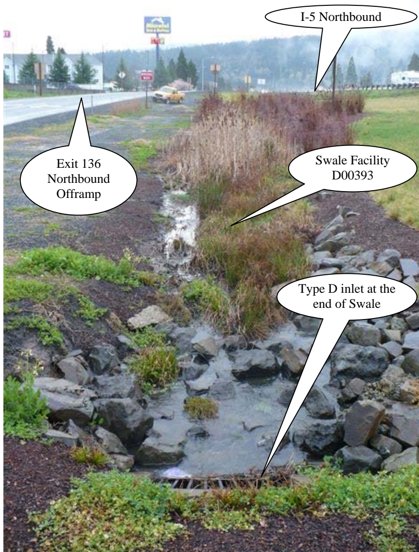
Photo 1: Looking south, flow into the swale is generated from a 15-inch storm pipe and sheet flow originating from the northbound travel lanes of I-5 and the Exit 136 northbound offramp. Water is flowing towards the bottom of the picture.
