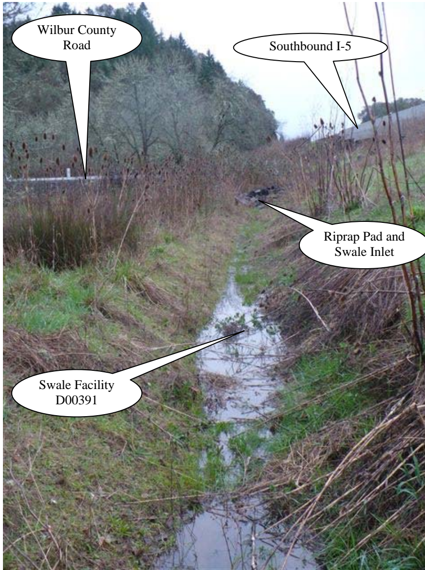
Photo 1: Looking north, flow into the swale is generated from the Wilbur Road overcrossing structures shown in the upper portion of the picture. Water is flowing towards the bottom of the picture.
