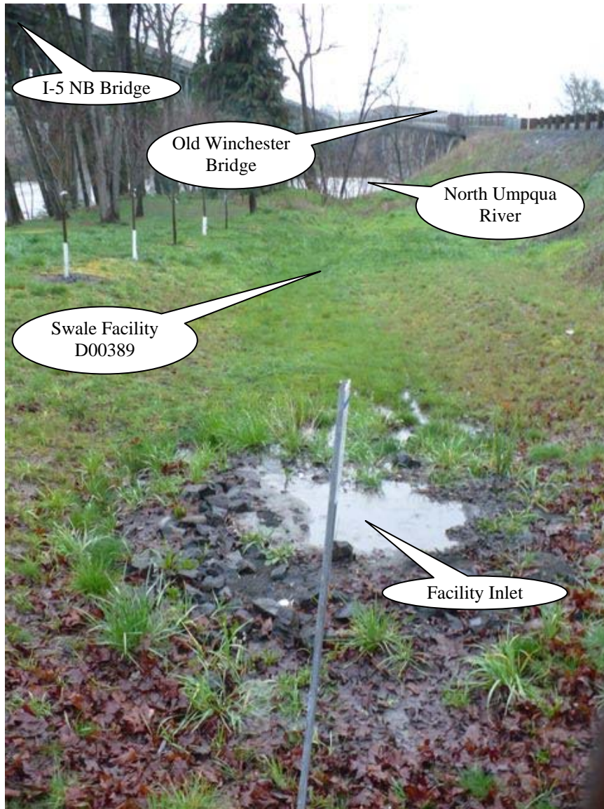
Photo 1: Looking north, flow into the swale is generated from the Old Winchester Bridge shown in the upper right portion of the picture. Water is flowing out of the Type G-2 inlet shown due to head pressure generated by the storm sewer system. The water is flowing towards the top of the picture and outfalls directly into the North Umpqua River.
