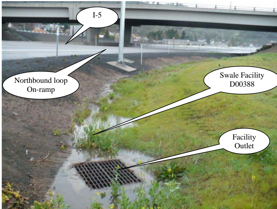
Photo 2: Looking north, flow into the swale is generated from the northbound loop on-ramp on the left side of the picture. Water is collected in the inlet/outlet structure shown at the bottom of the picture.
