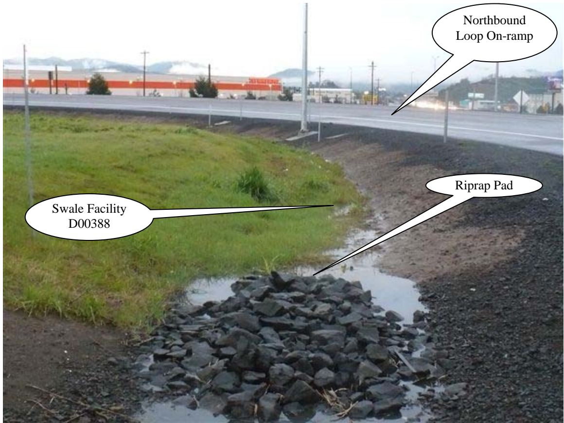
Photo 3: Looking east, flow into the swale is generated from the northbound loop on-ramp shown in the picture. Water is flowing towards the bottom of the picture.
