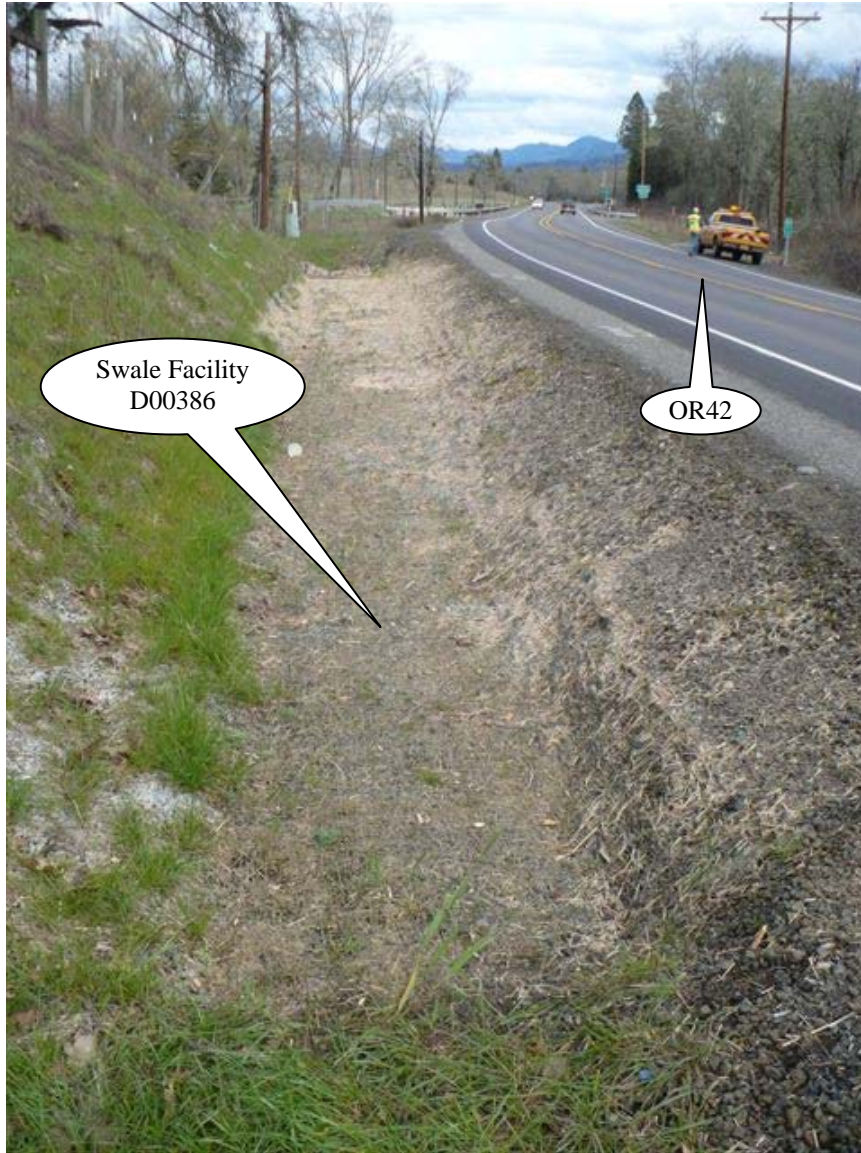
Photo 2: Looking east, sheet flow from OR42 on the right side of the picture contributes stormwater into the swale.
