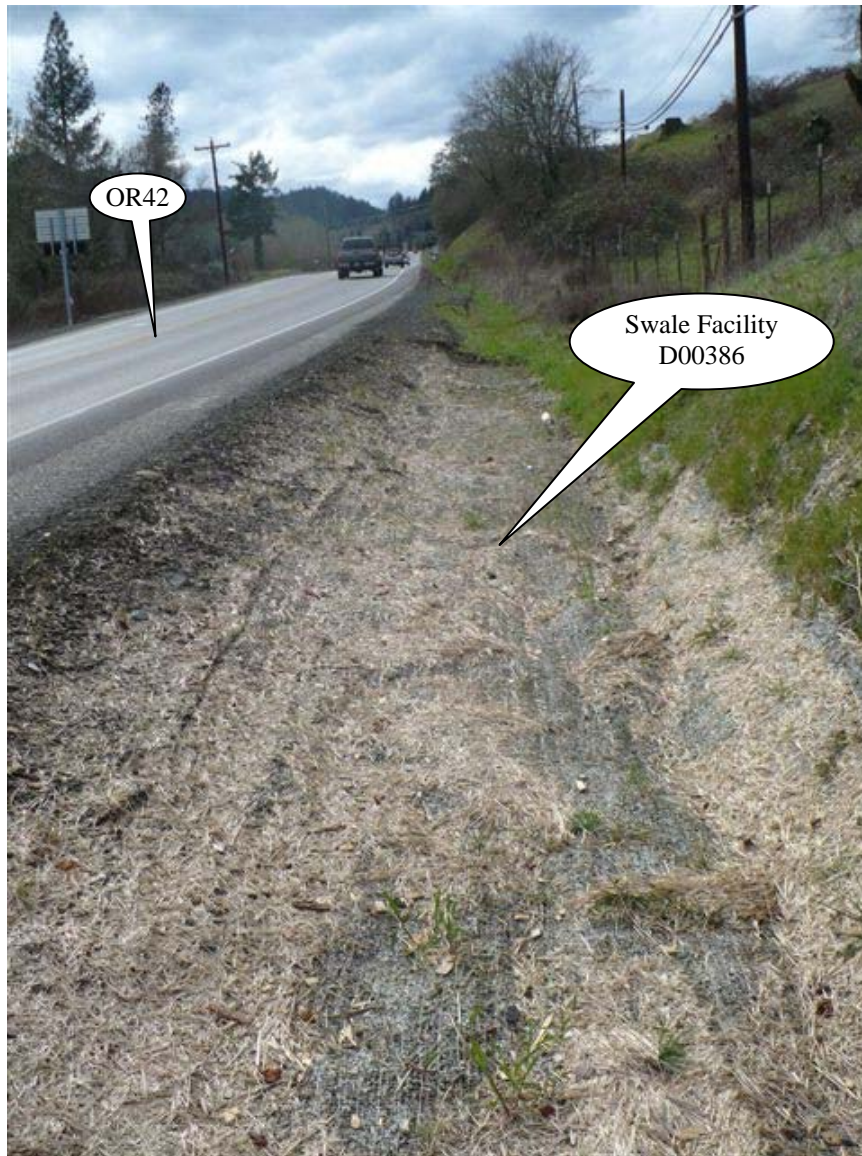
Photo 1: Looking west, sheet flow from OR42 on the left side of the picture contributes stormwater into the swale.
