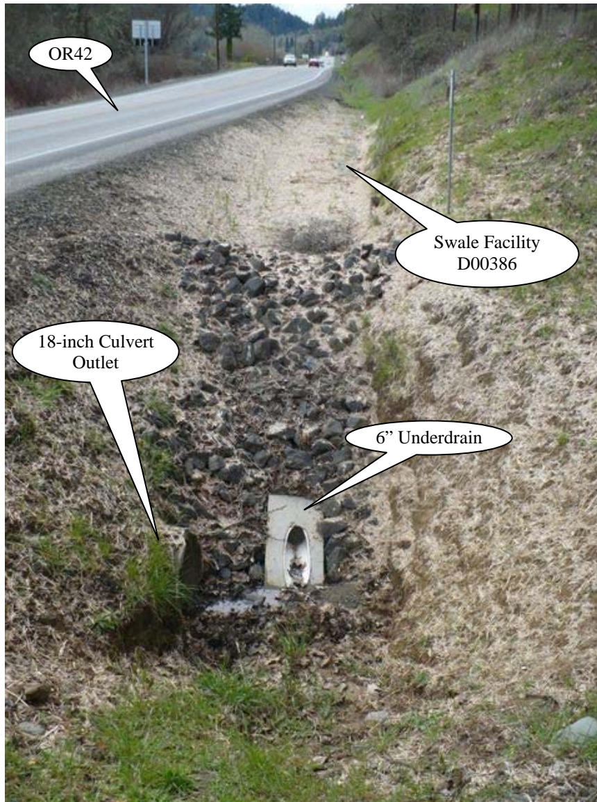
Photo 3: Looking west, flow from the swale and swale underdrain discharge directly into an 18" culvert.
