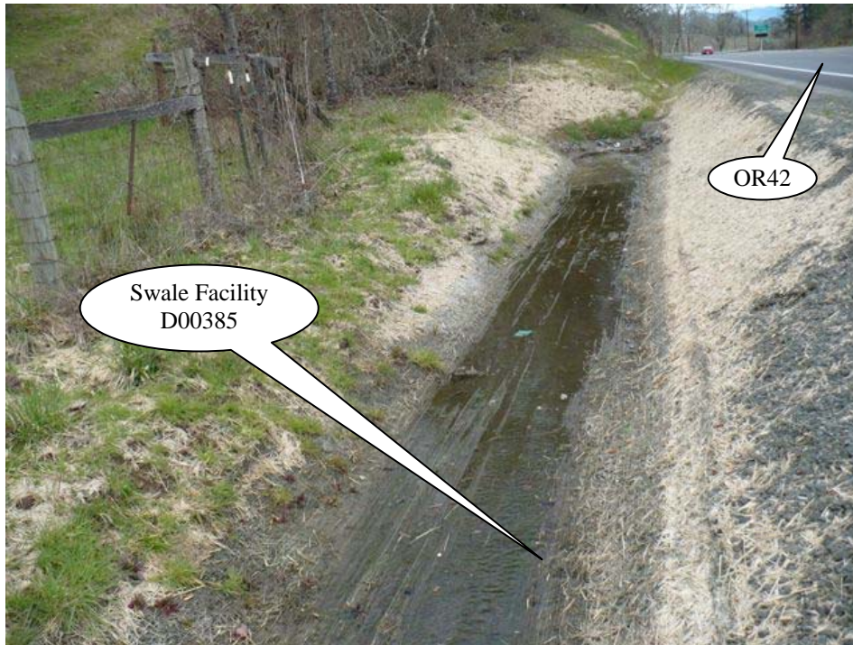
Photo 2: Looking east, sheet flow from OR42 on the right side of the picture contributes stormwater into the swale.
