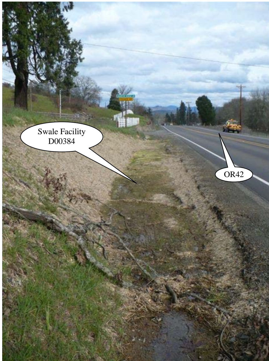
Photo 2: Looking east, sheet flow from OR42 on the right side of the picture contributes stormwater into the swale.
