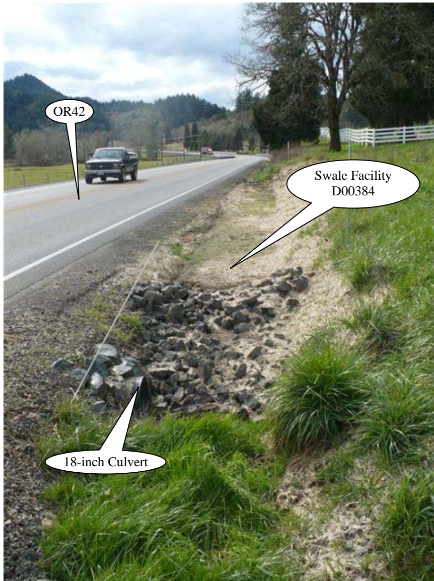
Photo 1: Looking west, sheet flow from OR42 on the left side of the picture contributes stormwater into the swale.
