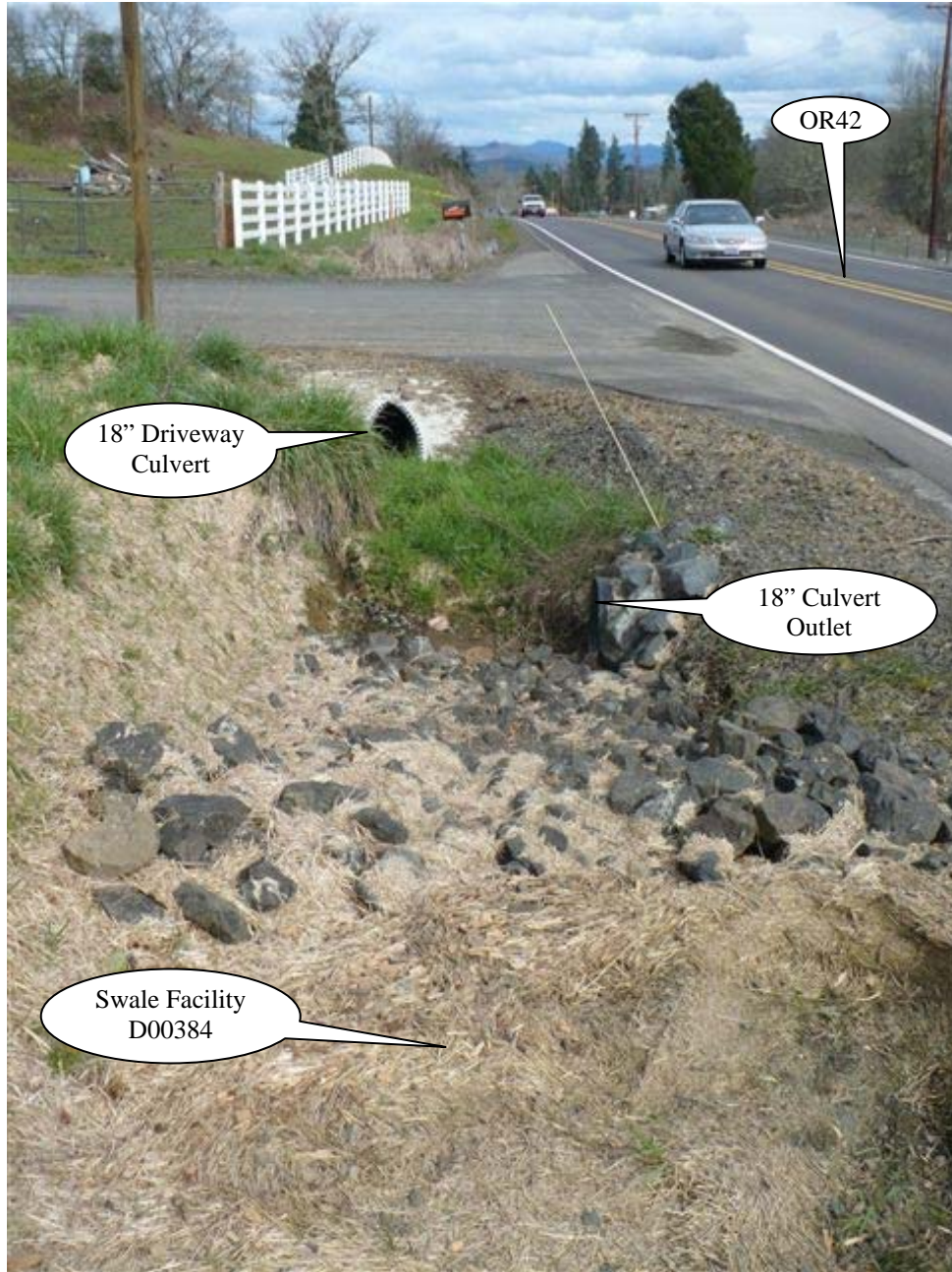
Photo 3: Looking east, flow from the swale discharges directly into an 18-inch culvert.
