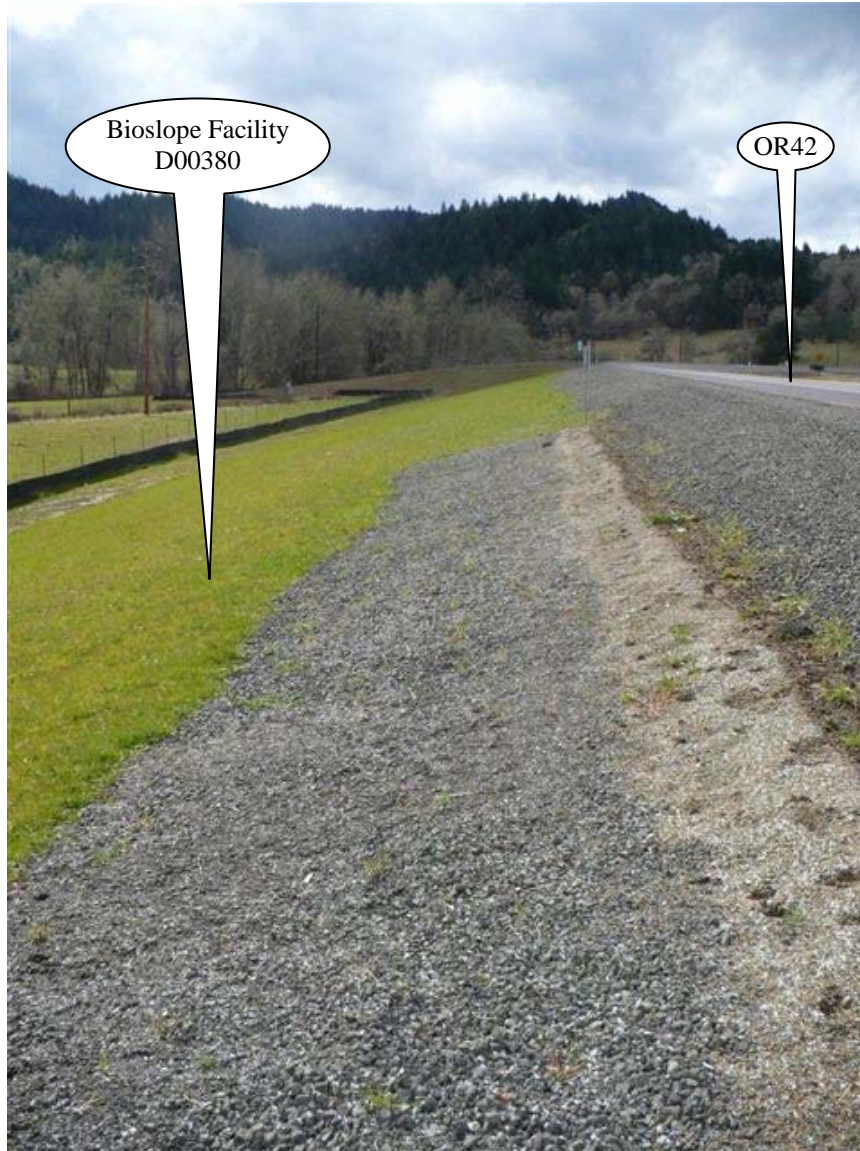
Photo 2: Looking west, sheet flow from OR42 on the right side of the picture contributes stormwater onto the bioslope.
