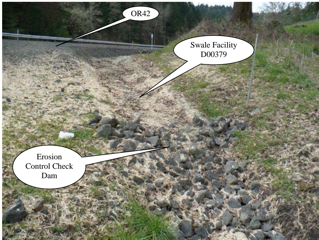
Photo 2: Looking west near the eastern-end of the facility. Sheet flow from OR42 on the left side of the picture contributes stormwater into the swale.
