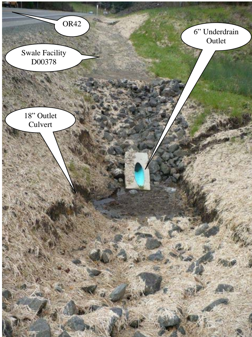
Photo 3: Looking west, flow into the swale is generated from OR42 on the left side of the picture.
