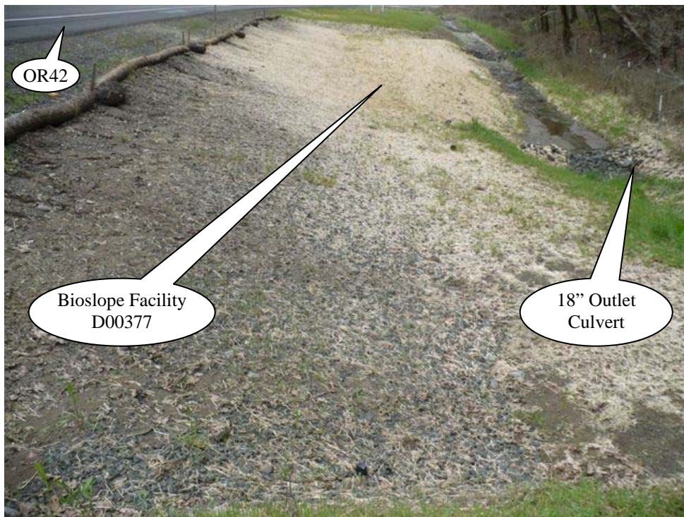
Photo 2: Looking west, sheet flow from OR42 on the left side of the picture contributes stormwater onto the bioslope.
