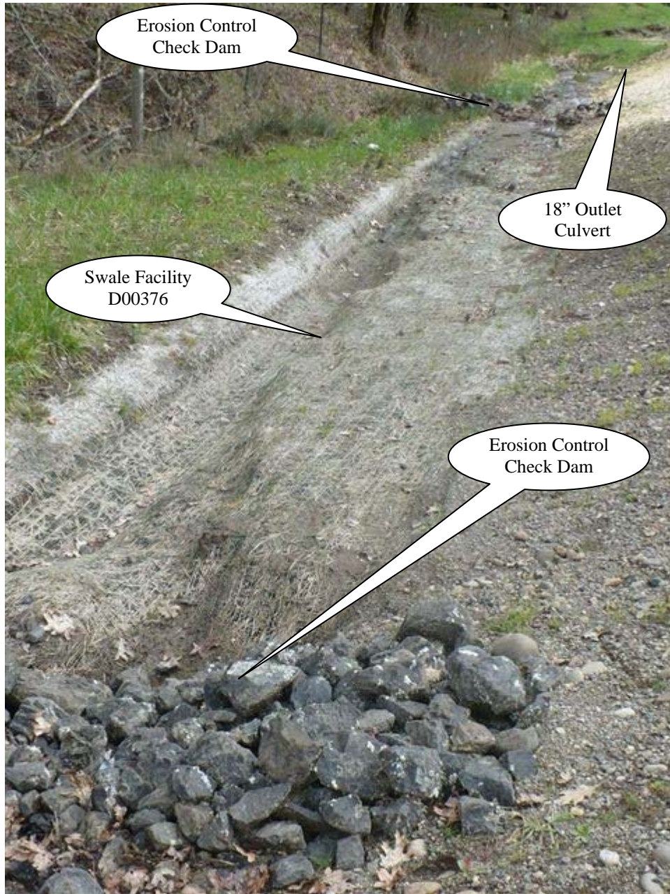
Photo 3: Looking east, flow into the swale is generated from OR42 on the right side of the picture.
