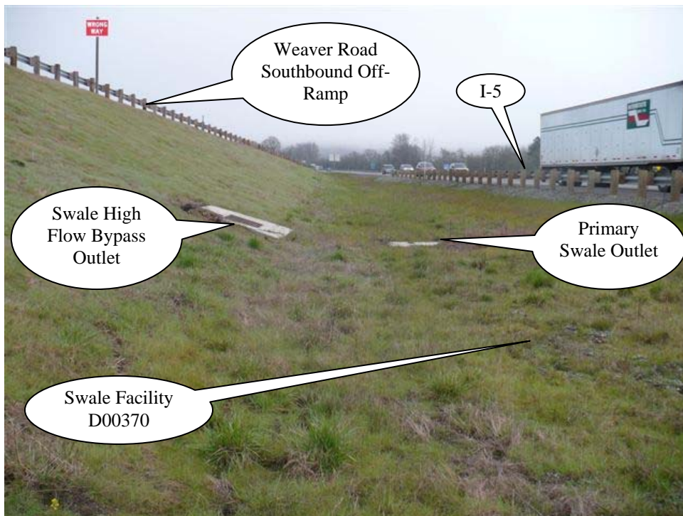
Photo 2: Looking north, flow into the swale is generated from I-5 shown on the right side of the picture and from the Weaver Road off-ramp shown to the left.
