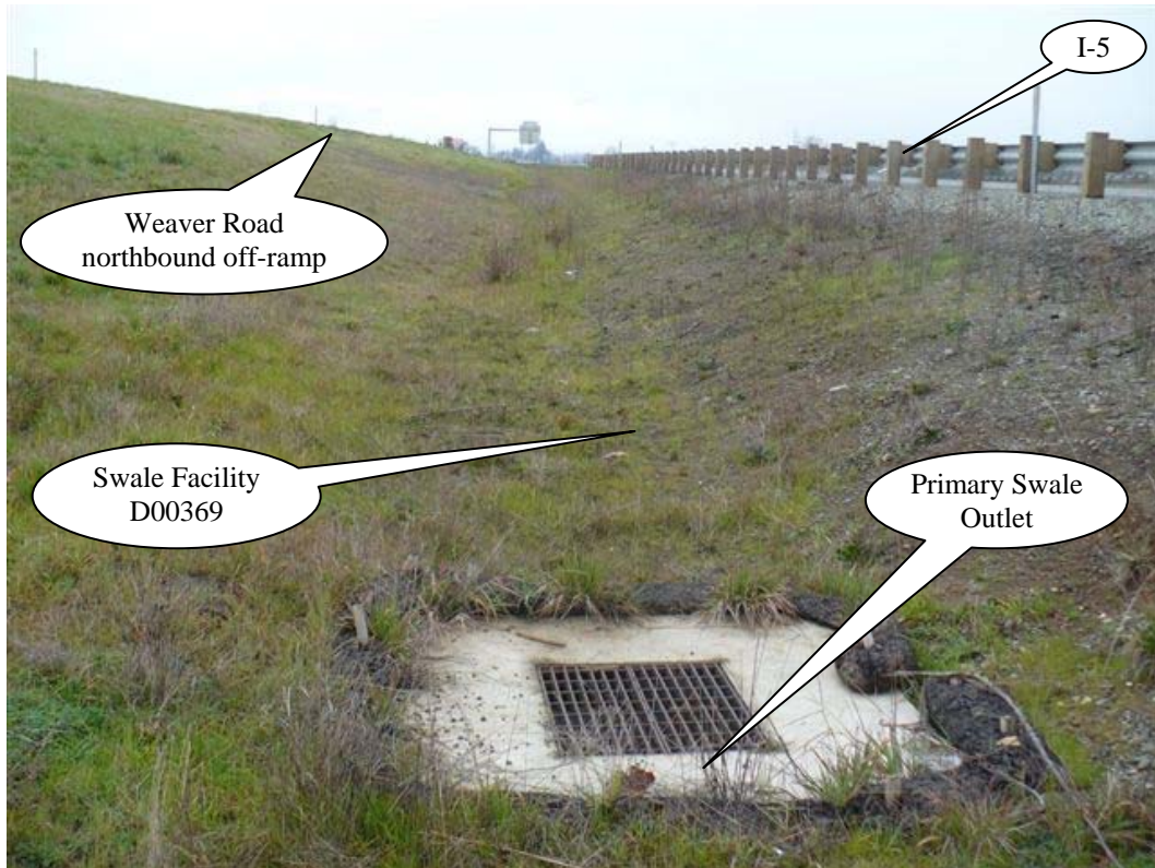
Photo 3: Looking south, flow into the swale is generated from I-5 shown on the right side of the picture and from the Weaver Road NB off-ramp shown to the left.
