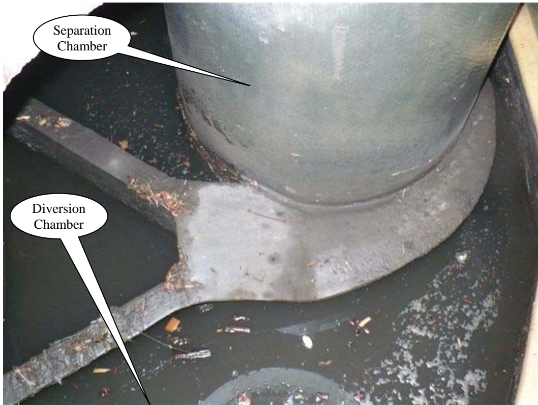
Photo 2: Interior of water quality manhole DFI D00368.
