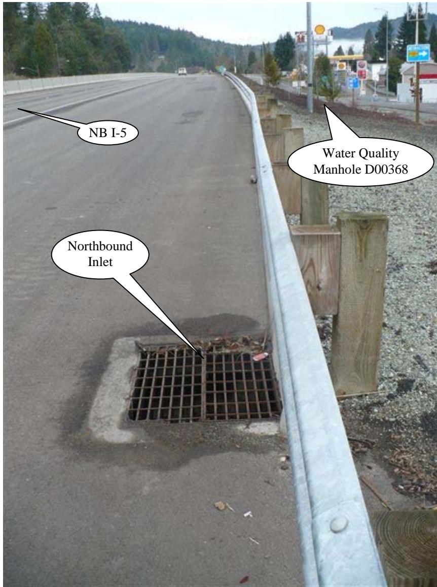
Photo 3: Looking north with, the northbound collection inlet shown in the foreground. Flow is conveyed directly from this inlet to the water quality manhole shown in the upper right portion of the picture.
