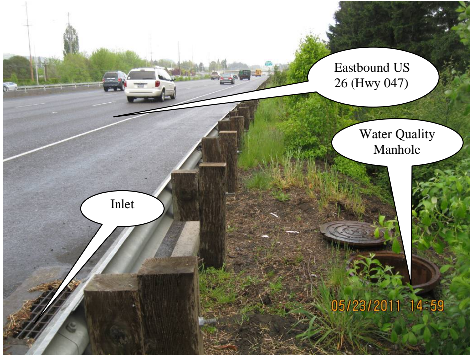
Photo 1: Water Quality Manhole looking eastbound on US 26 (Hwy 047).
