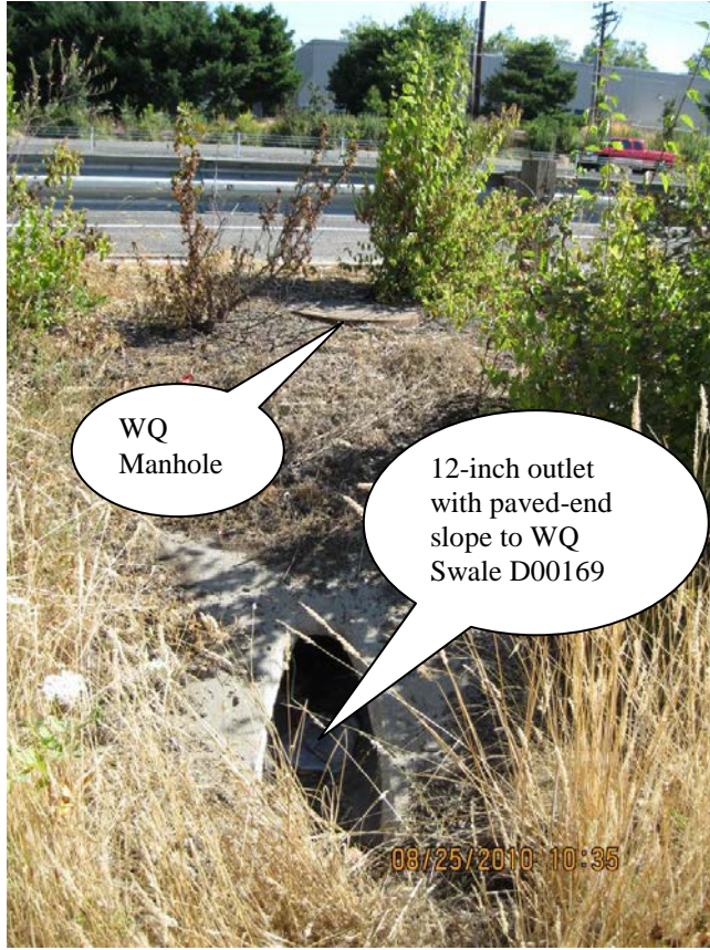
Photo 1: Exterior view of Water Quality Manhole structure.
