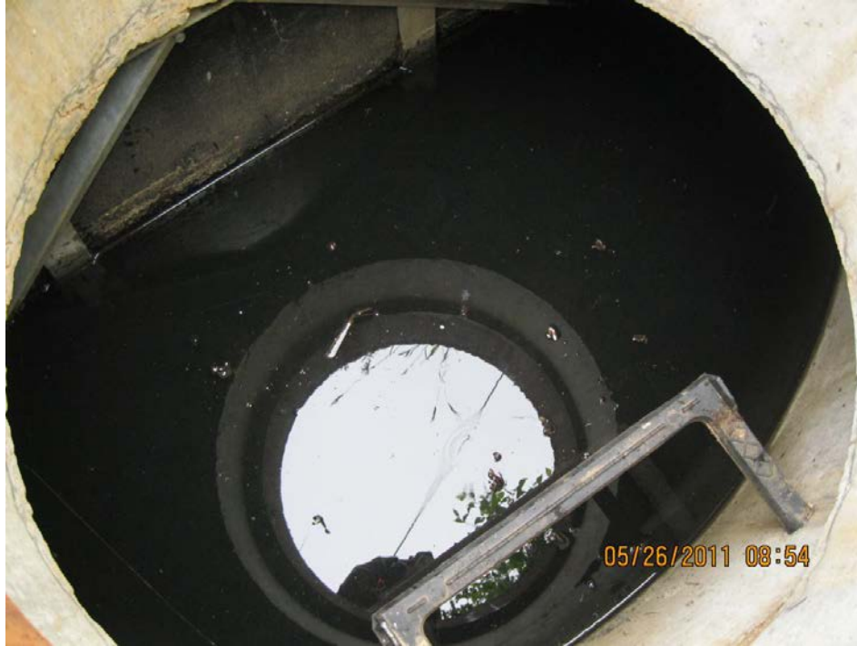
Photo 2: Interior view of Water Quality Manhole structure.
