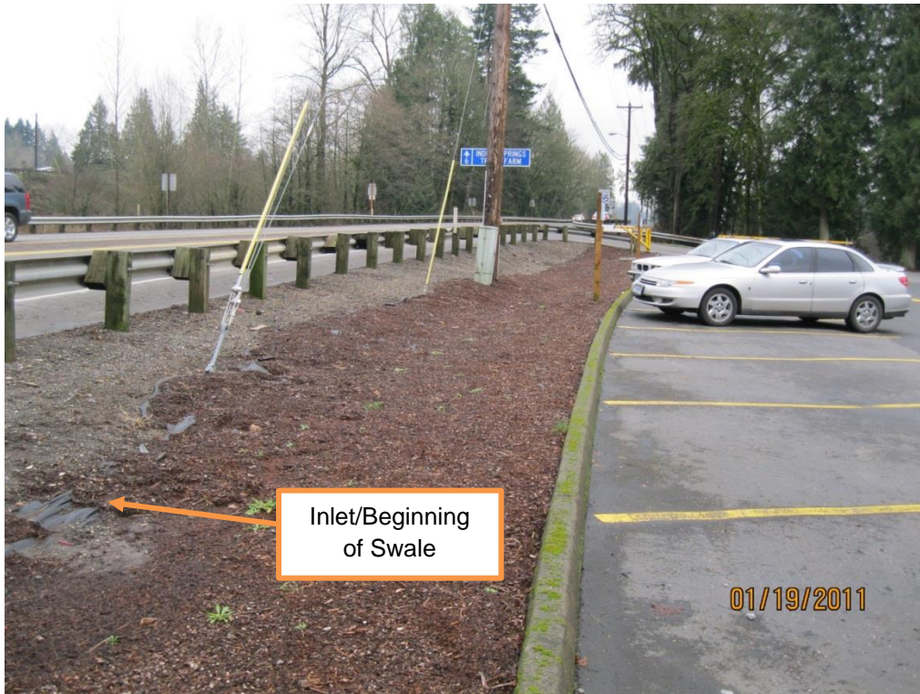
Figure 3: Facility access via adjacent parking lot
