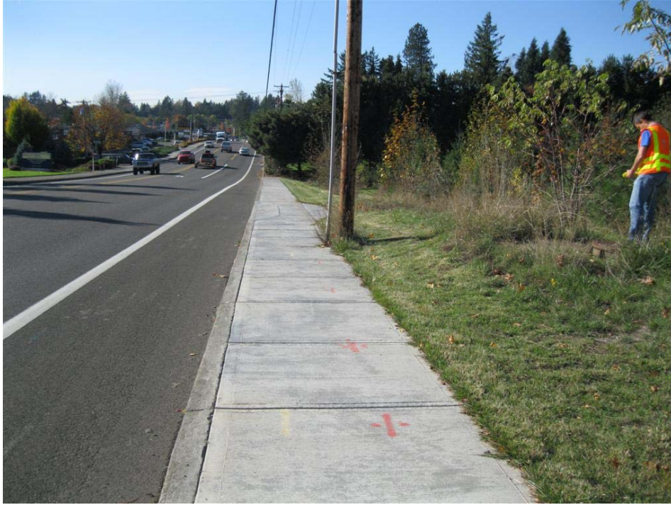
Photo 2: Pond/Swale Combo facility looking west toward the facility inlet and maintenance access pad. Hwy 174 is located to the left.
