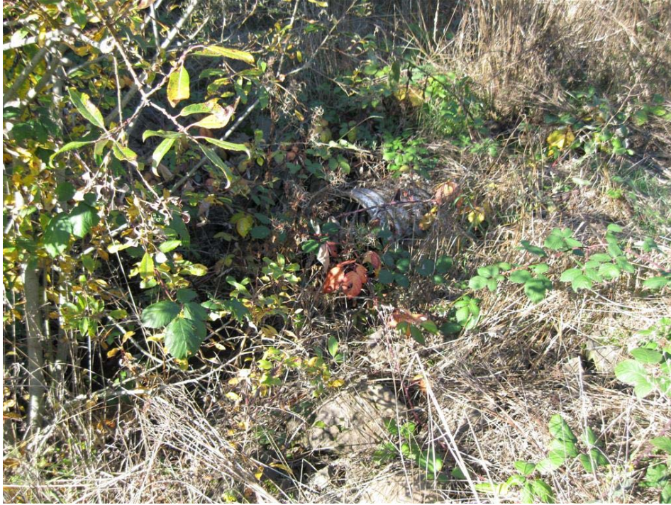
Photo 4: Looking north at the outlet pipe (Point D) of the Pond/Swale Combo facility.
