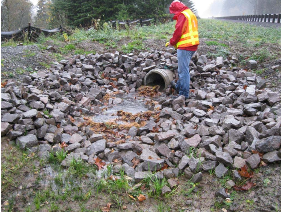
Photo 1: Water Quality Biofiltration Swale, looking east at the facility inlet. I-84 is located to the right.
