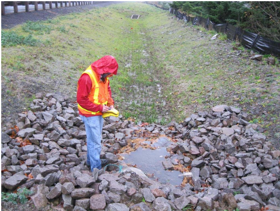
Photo 2: Water Quality Biofiltration Swale, looking west. I-84 is located to the left.
