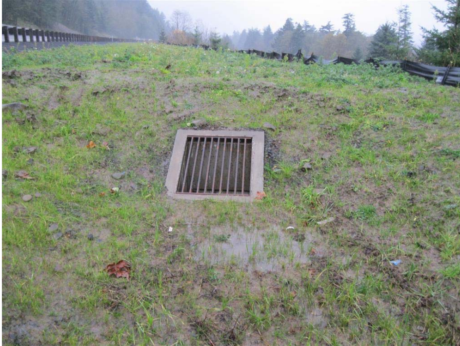
Photo 3: Water Quality Biofiltration Swale, looking west at the facility outlet. I-84 is located to the left.
