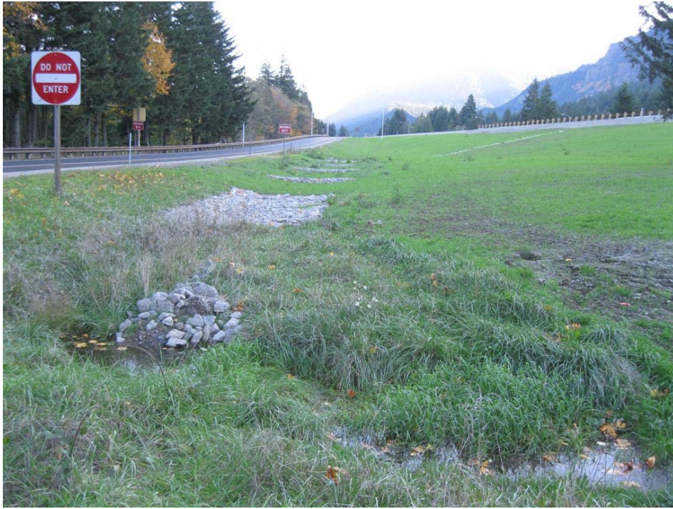
Photo 4: Water quality facility outfall to ditch looking east. Off-ramp located to the left.
