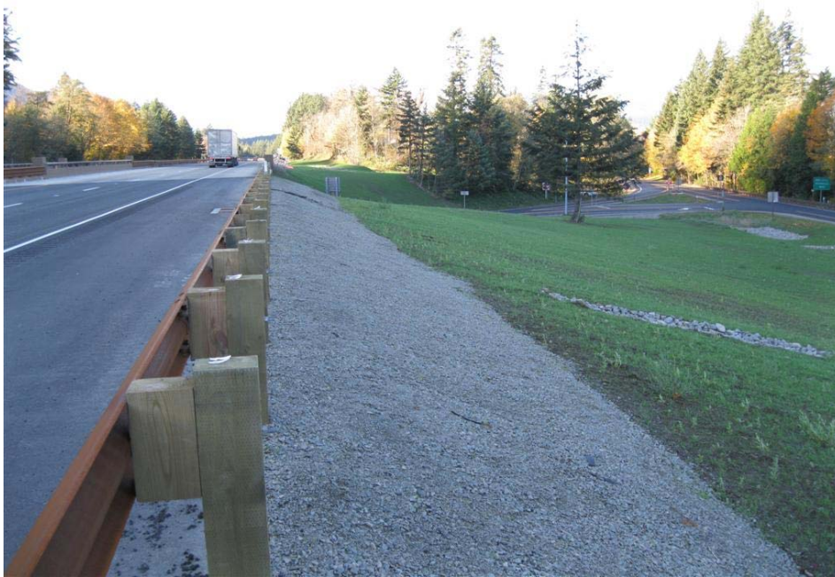
Photo 1: Looking west. Water quality facility, below, to the right with I-84 on the left.
