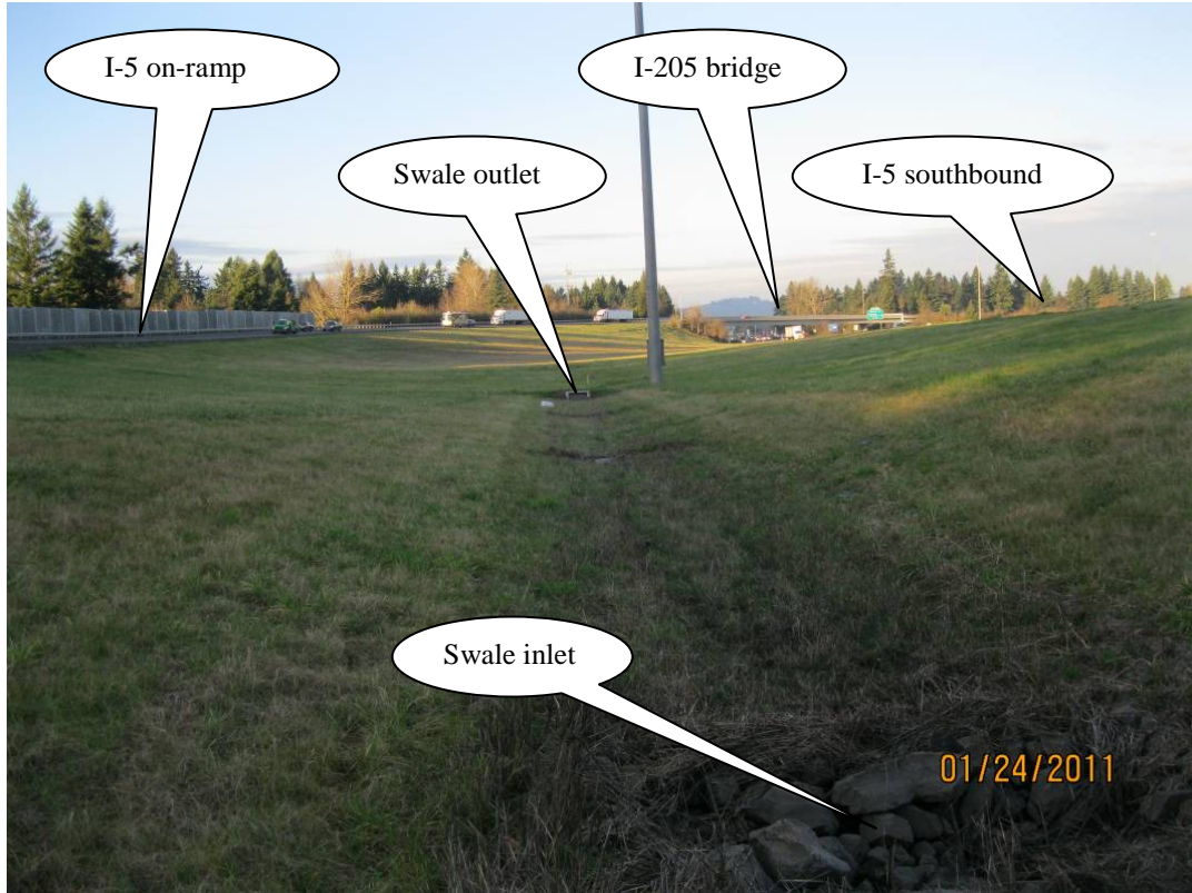
Photo 1: Water Quality Biofiltration Swale looking north
