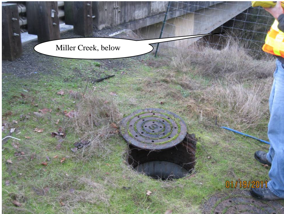
Photo 1: Looking southeast toward the manhole with the highway on the left.
