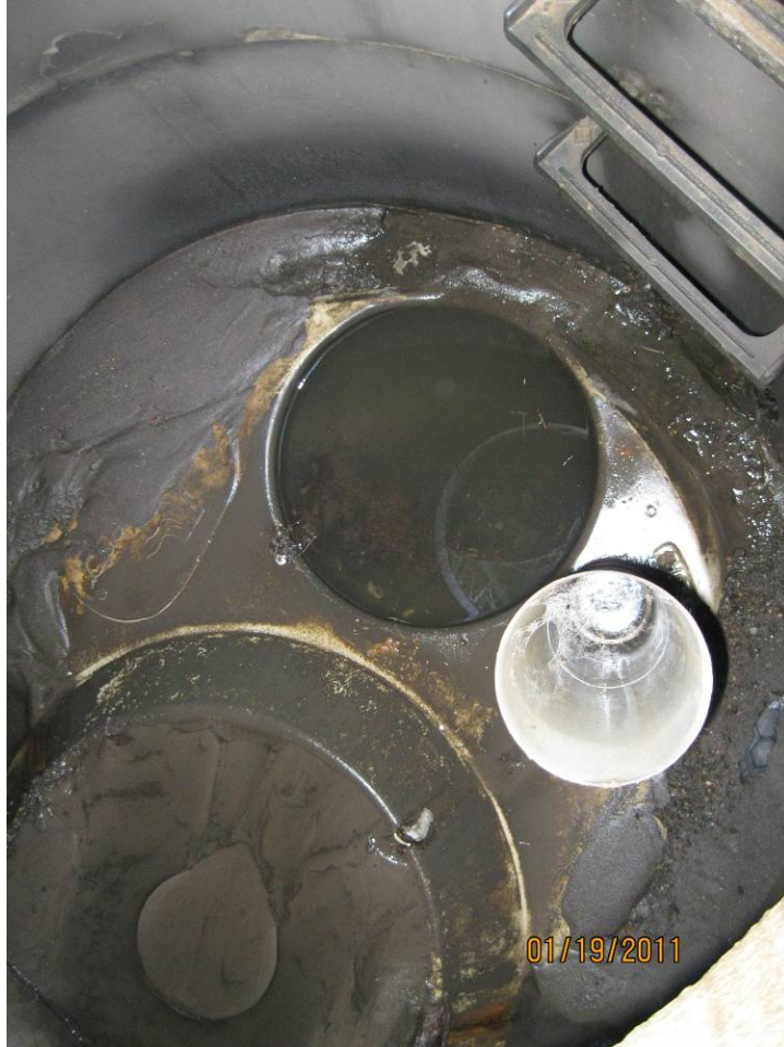
Photo 3: Interior view of the water quality manhole (CDS Unit)
