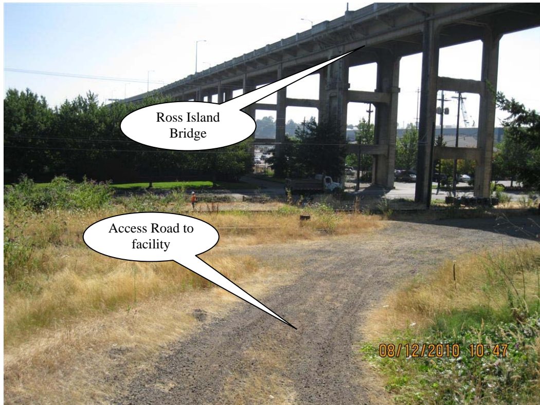
Photo 7: Gravel access road to facility. Photograph is looking towards the southeast at the Ross Island Bridge (US 026).
