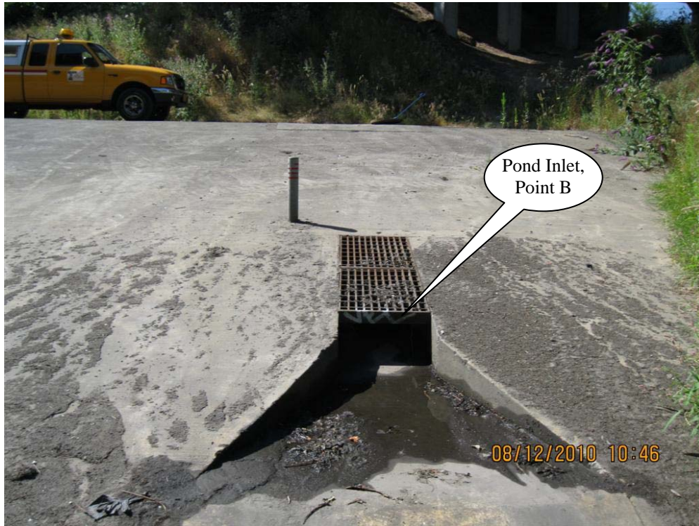
Photo 3: Close up of pond inlet. Pretreated water from a water quality manhole (DFI D00288) is directed into this inlet. Notice the fine sediment buildup.
