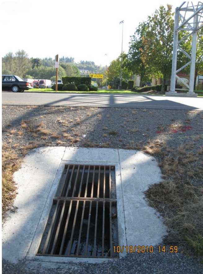
Photo 2: Outlet structure at Point B, looking south.
