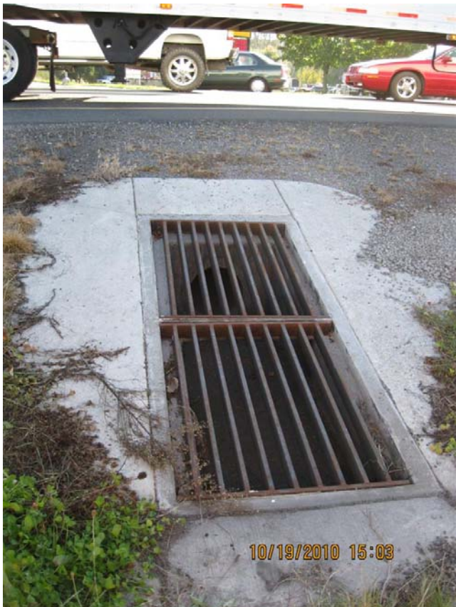
Photo 4: Outlet structure at Point A, looking south.
