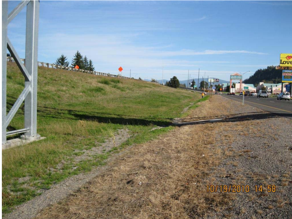
Photo 1: Water Quality Biofiltration Swale, looking east. I-84 is located to the left; NW Frontage Road to the right.
