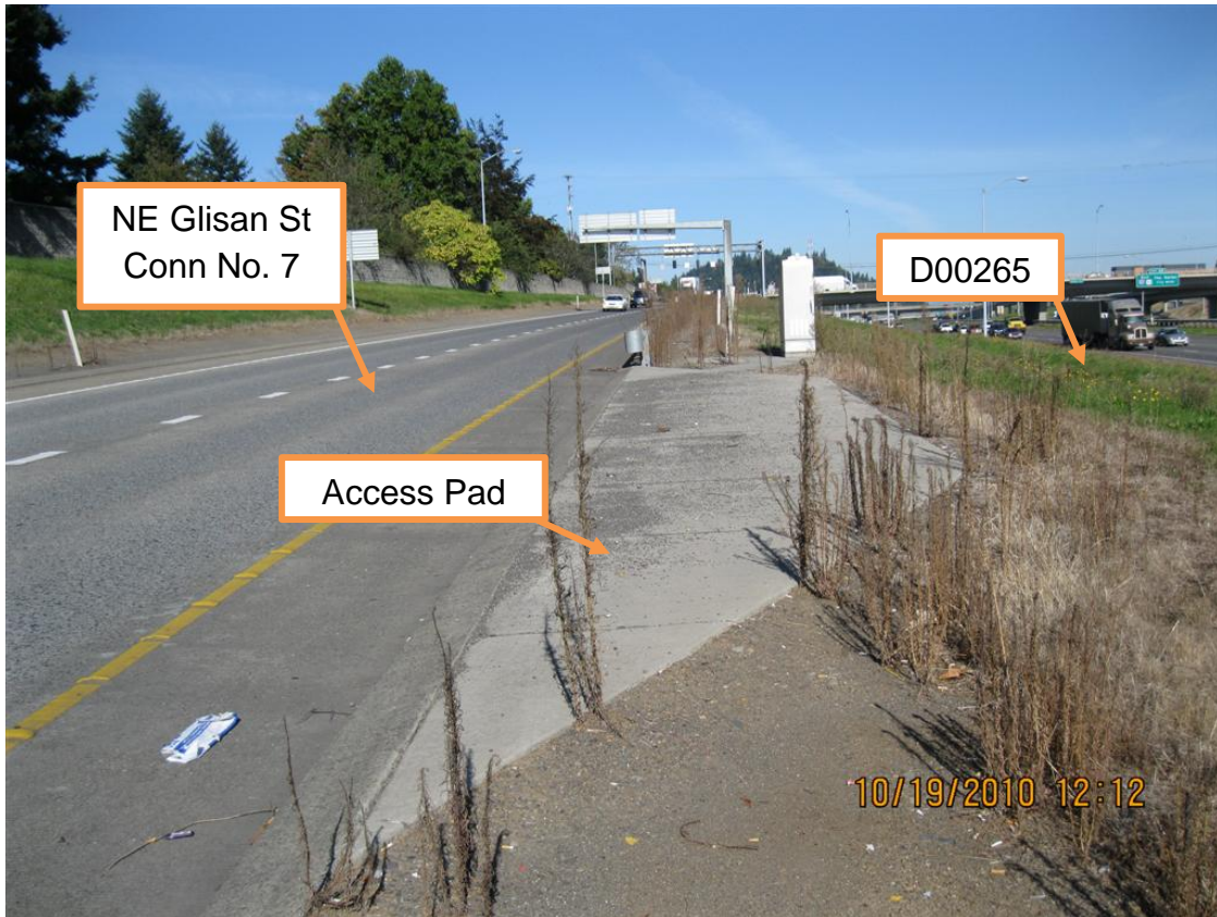
Figure 3: Facility access pad, looking North
