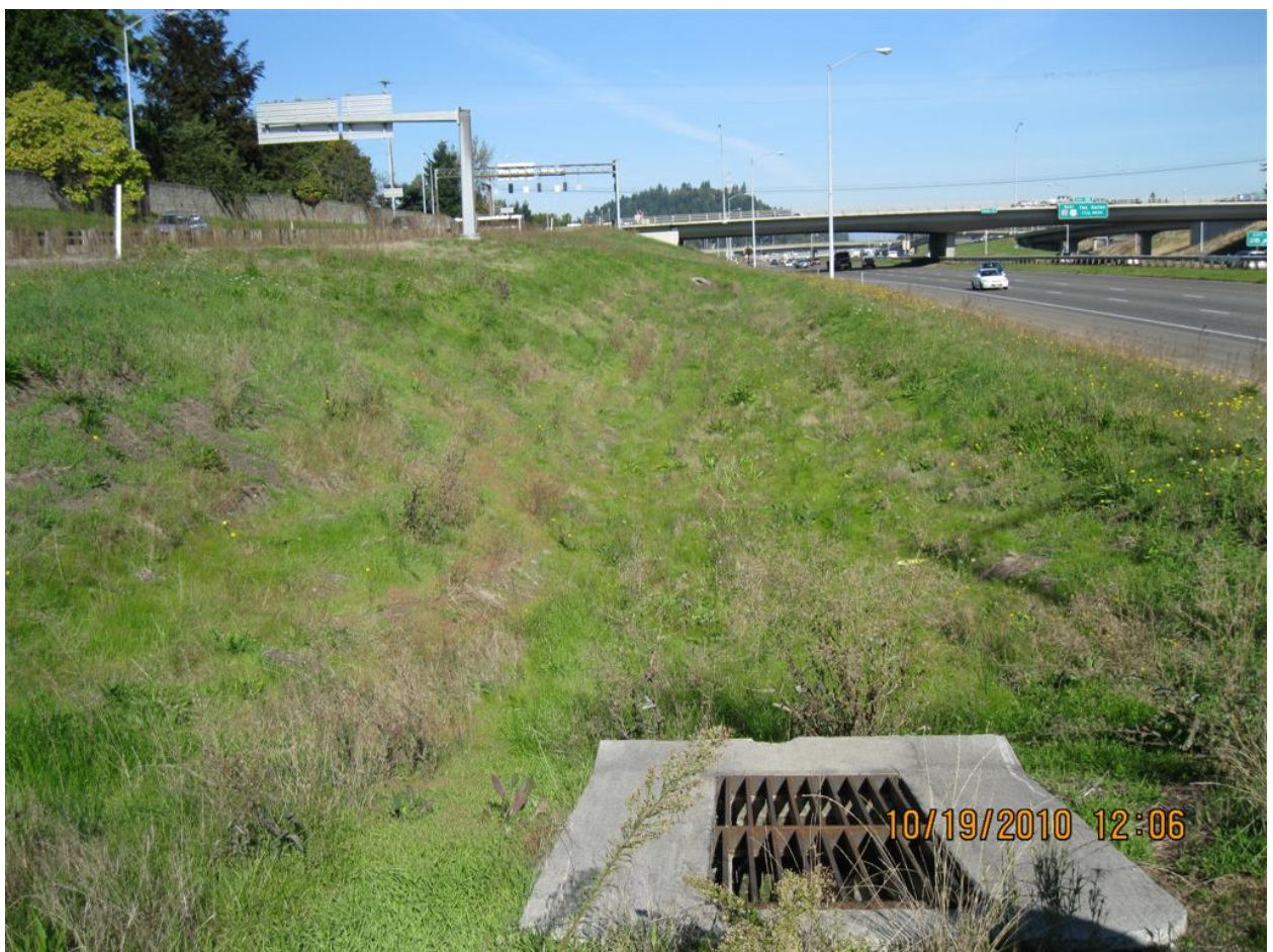
Figure 1: DFI No. D00265, looking North
