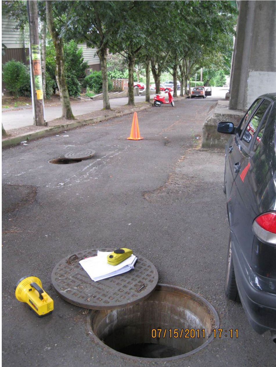
Photo 1: Looking south at water quality manhole (nearest). While plans only showed one manhole near bridge pier, it is apparent two are present. A downstream standard manhole is shown in the background.
