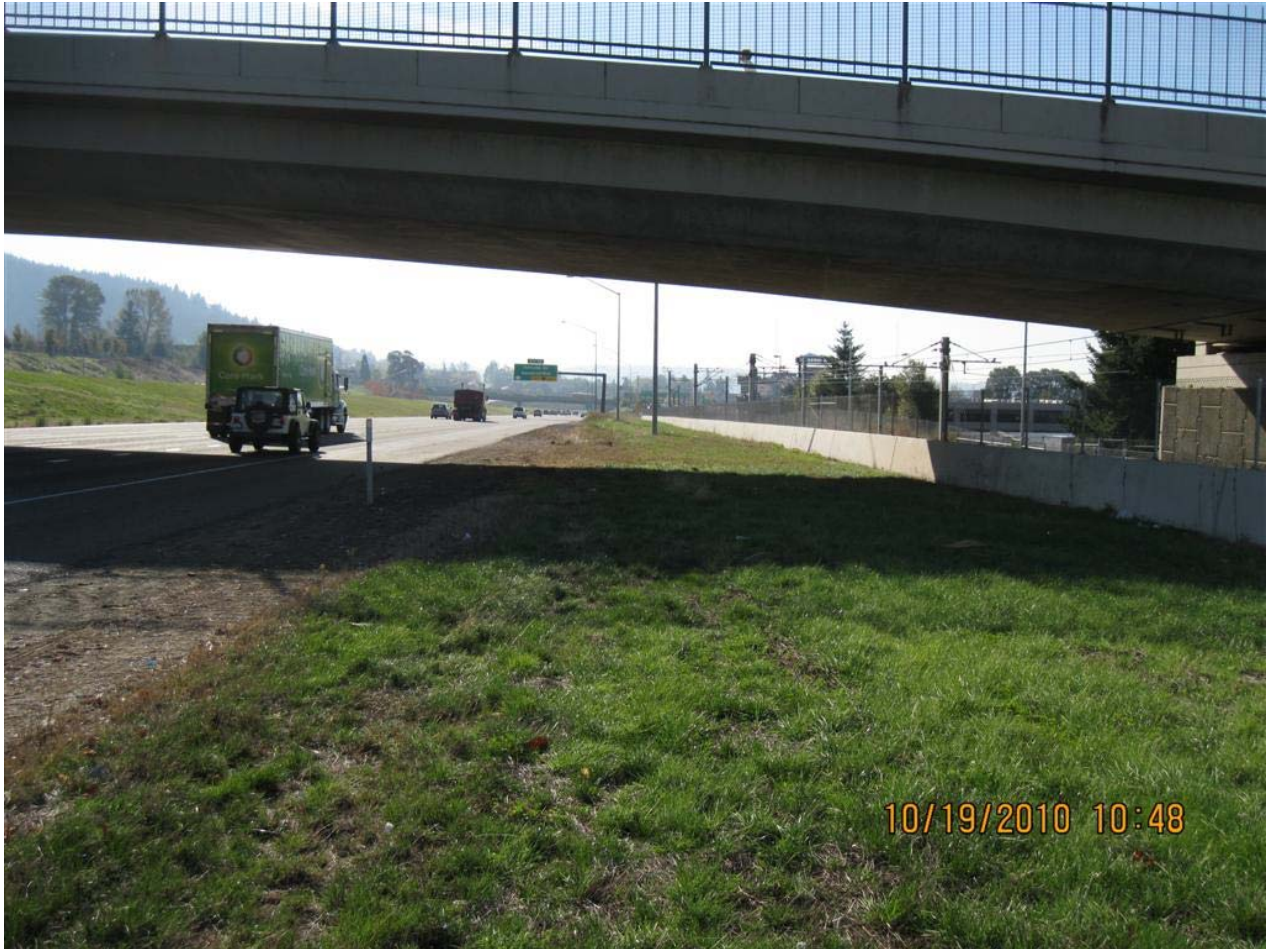
Figure 3: Swale footprint with shoulder access, looking south
