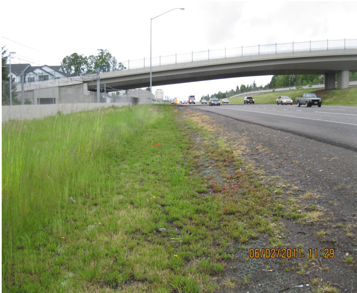
Figure 1: DFI No. D00255, looking north
