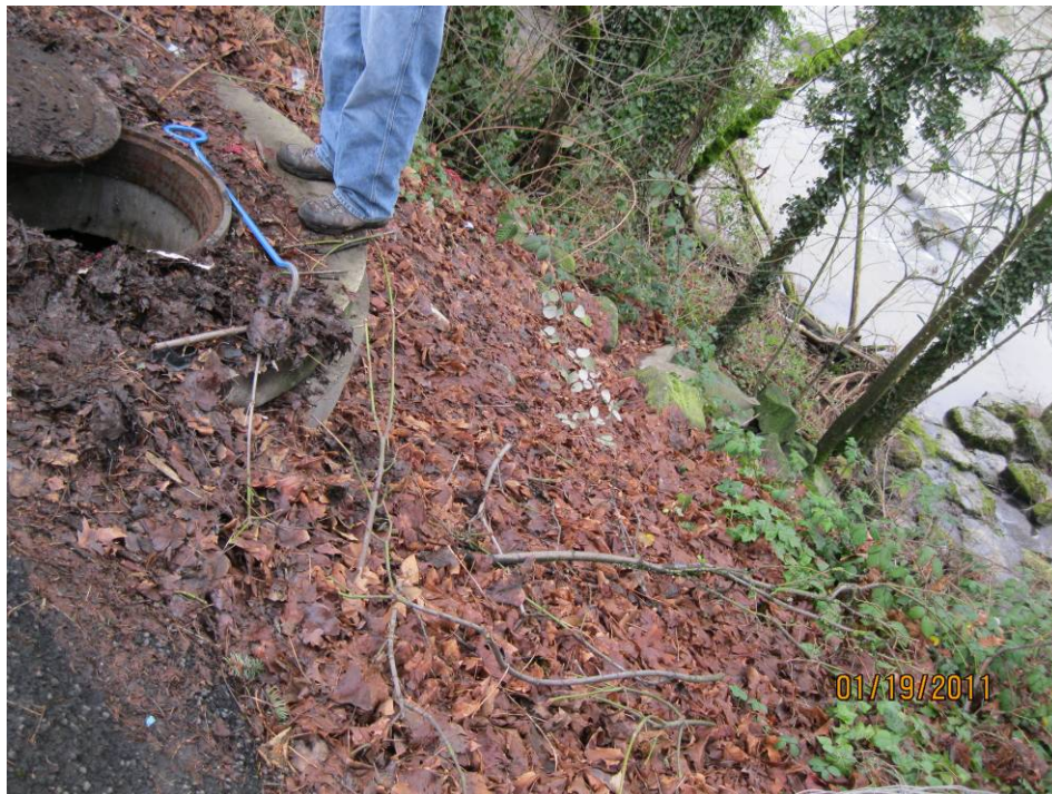
Photo 4: View of WQ manhole and rock-lined outfall, below, along Clackamas River.
