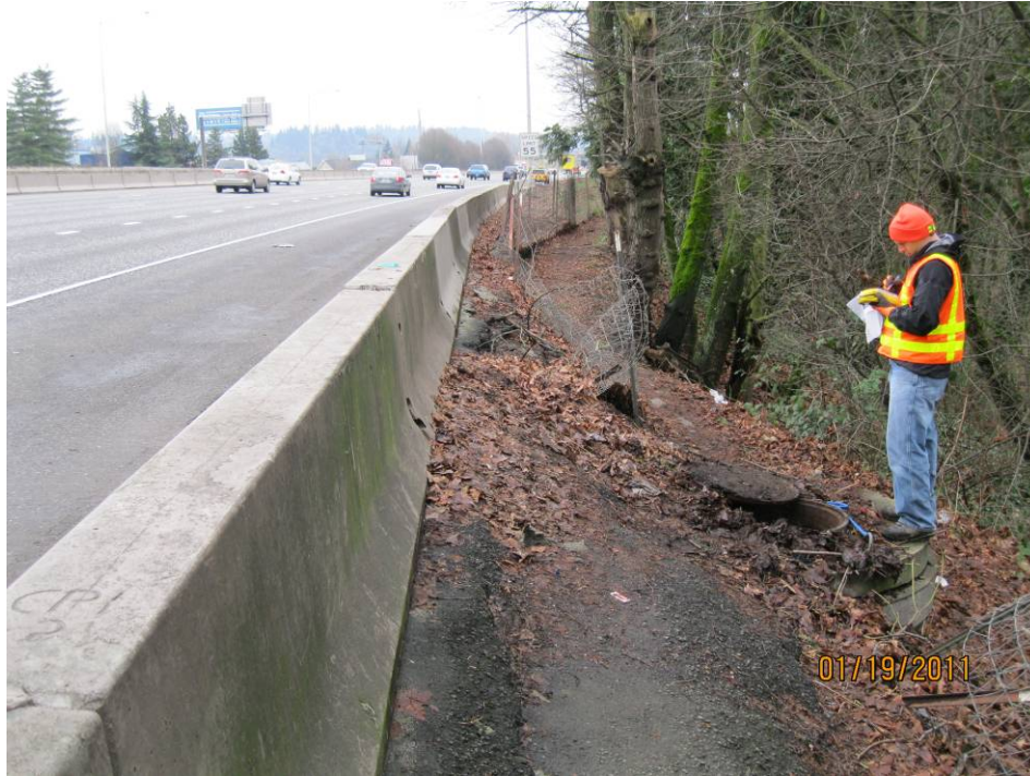
Photo 1: Looking south at water quality manhole. SB I-205 is located to the left.
