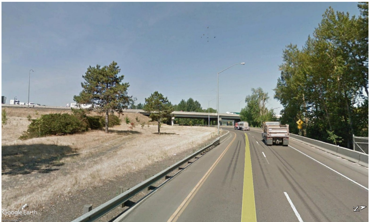
Figure 1: DFI No. D00249, looking West
