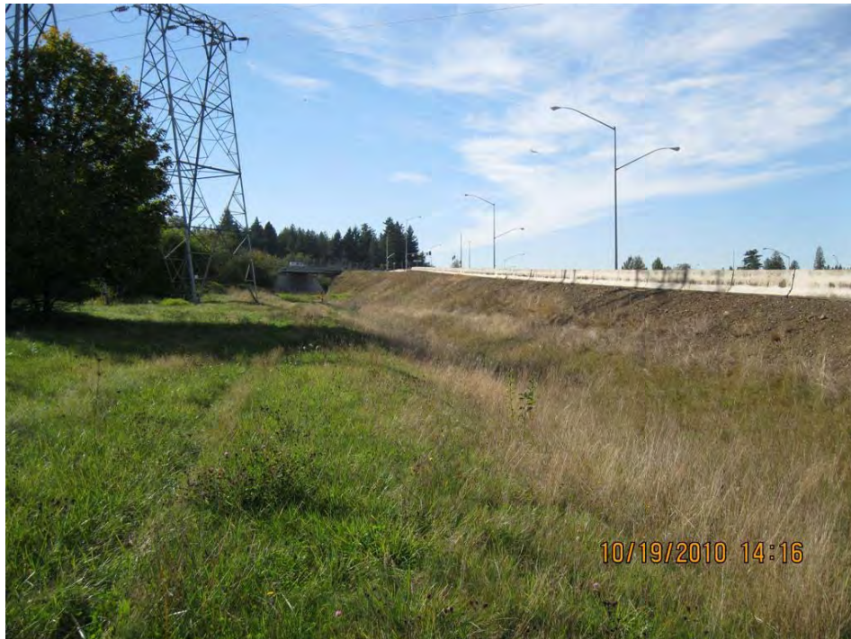
Photo 2: Looking west toward the facility inlet and on-ramp. The ramp and I-84 are located to the right.
