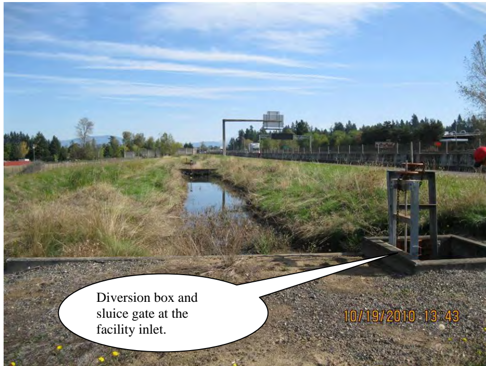
Photo 2: Detention Pond Facility, looking east. Diversion box (sediment vault), sluice gate and headwall at the facility inlet; Points A and B.
