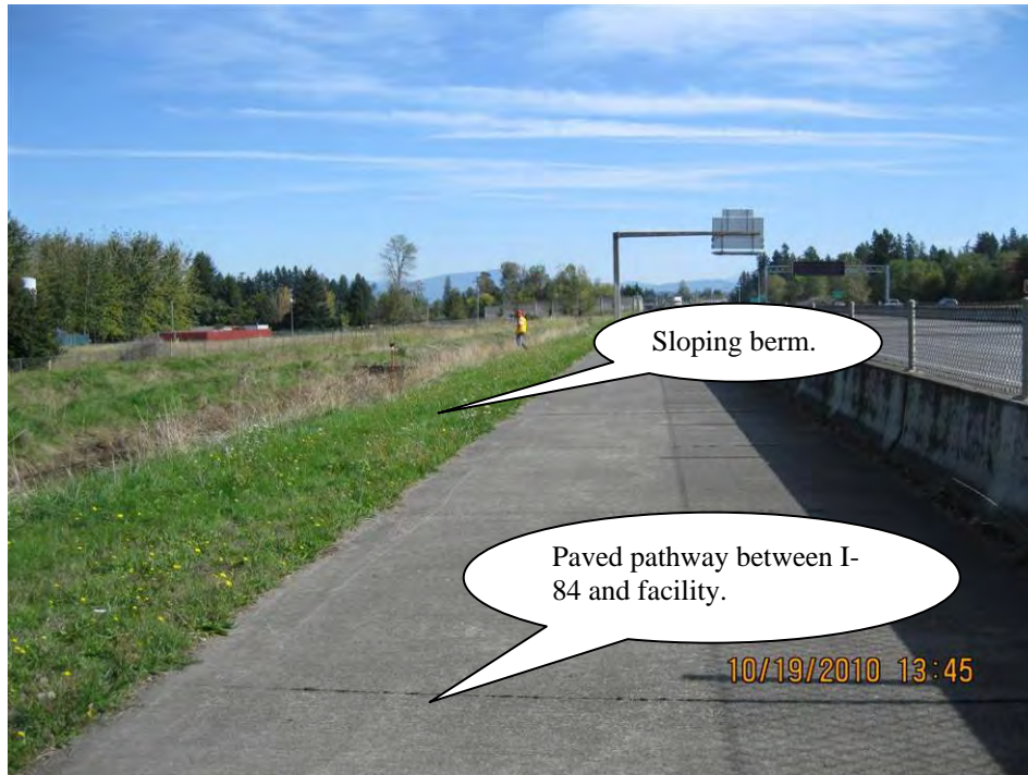
Photo 1: Detention Pond Facility on left, looking east. I-84 is located to the right.
