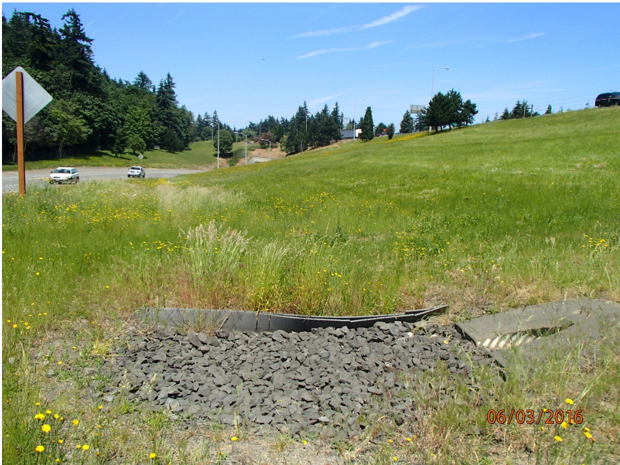
Figure 1: DFI No. D00242, looking North
