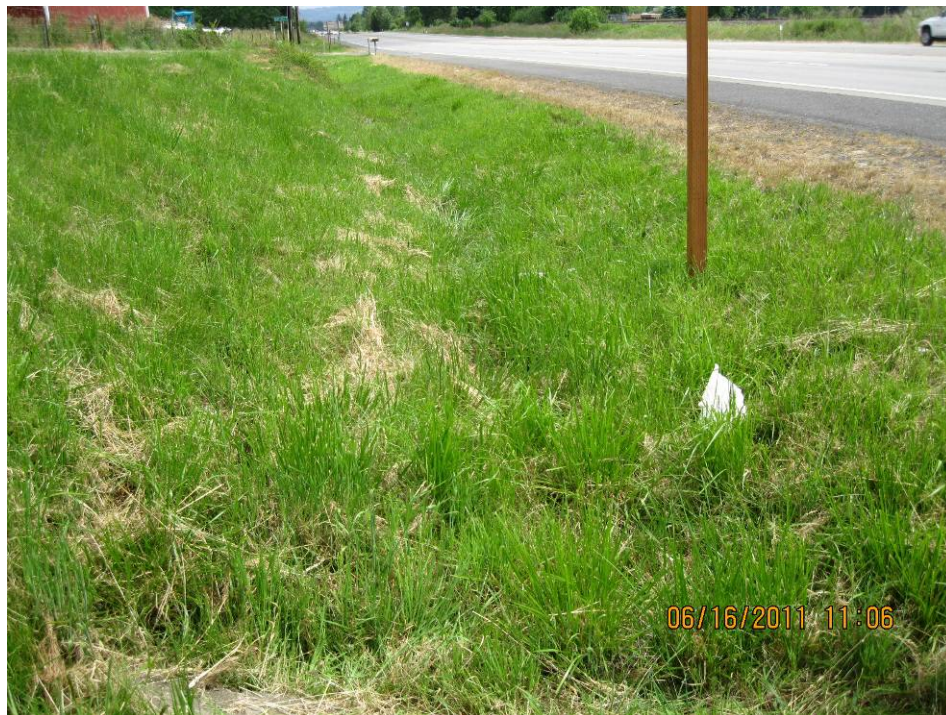
Photo 2: Looking north at water quality swale near the swale entrance. Hwy 92 is located to the right.
