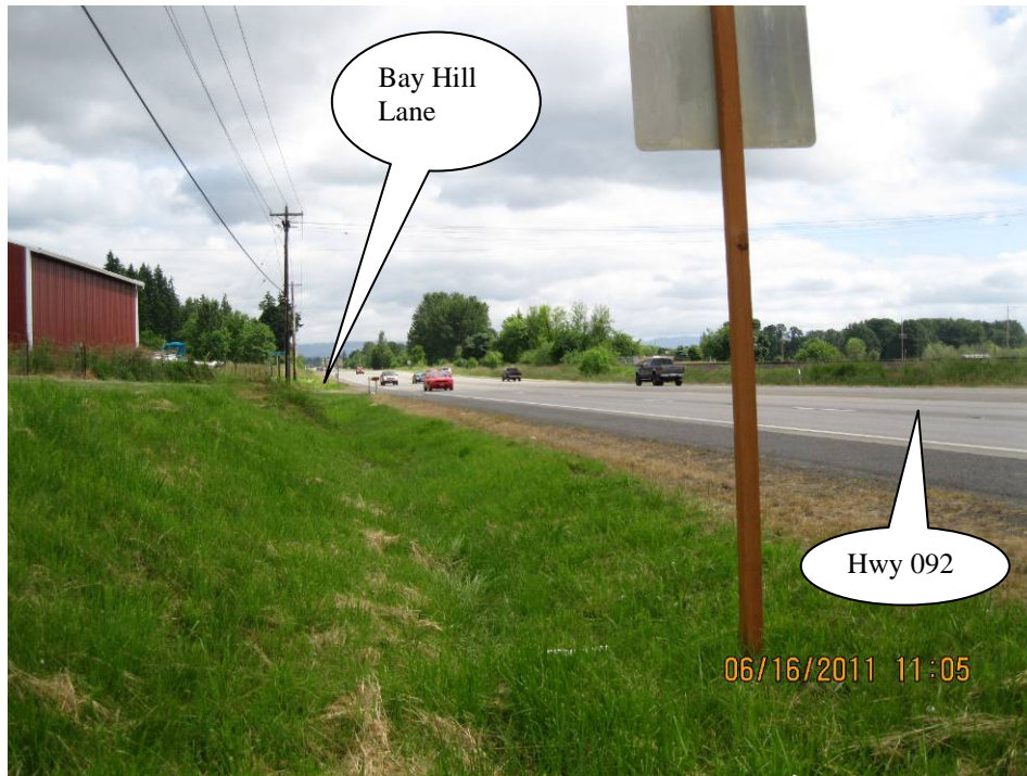
Photo 1: Looking north at water quality swale. Hwy 92 is located to the right.
