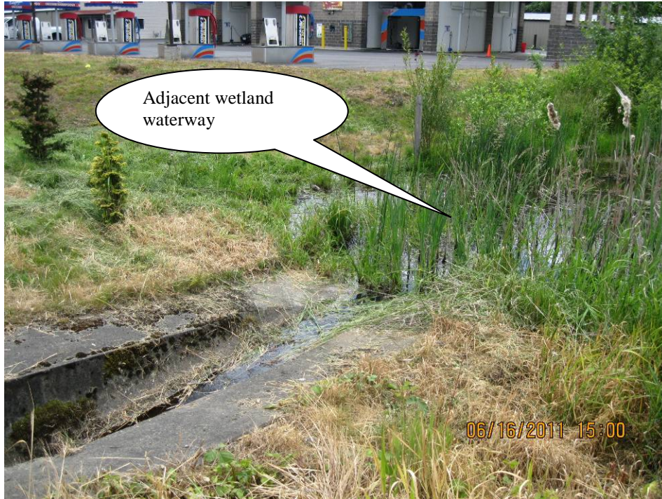
Photo 5: Looking west toward the wetland water source and culvert entrance/paved-end slope near the middle of the swale.
