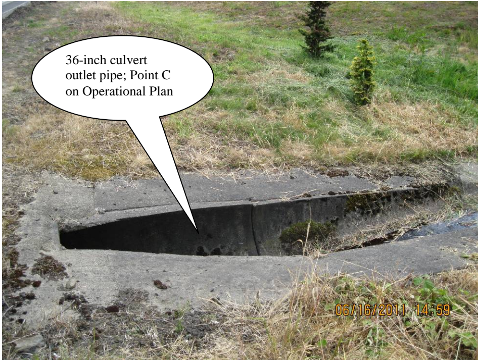
Photo 4: Looking south at the culvert entrance/paved-end slope near the middle of the swale.
