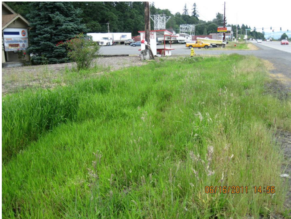
Photo 2: Looking north toward the beginning of the swale.
